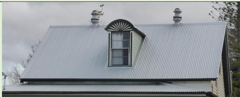
Zincalume roof on left hand side compared to galvanised roof on right hand side.
