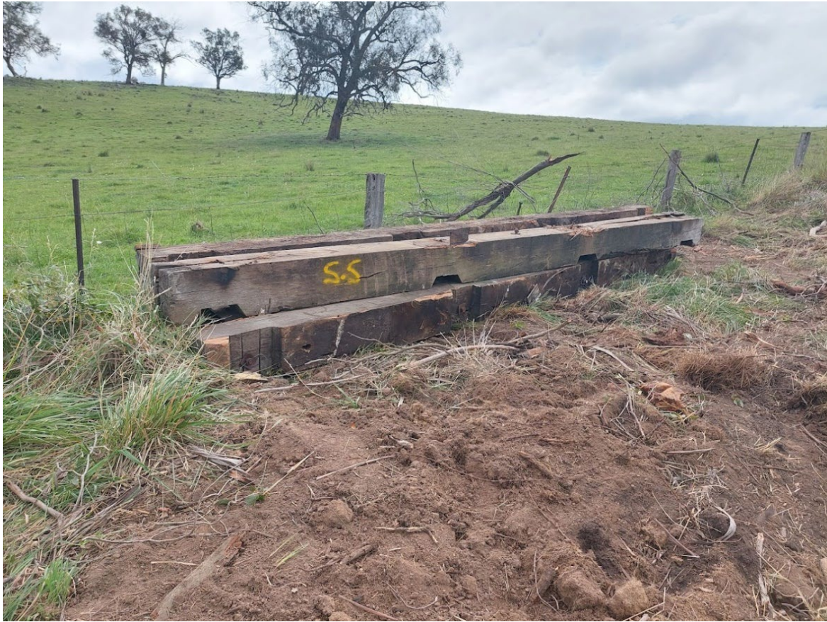
Figure 5 & 6 : Bridge headstocks, 300 x 300mm x 5.5m long
