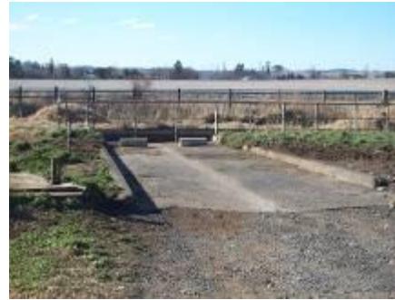
Photos 5 and 6: Truck wash and sediment trap for sales yard
