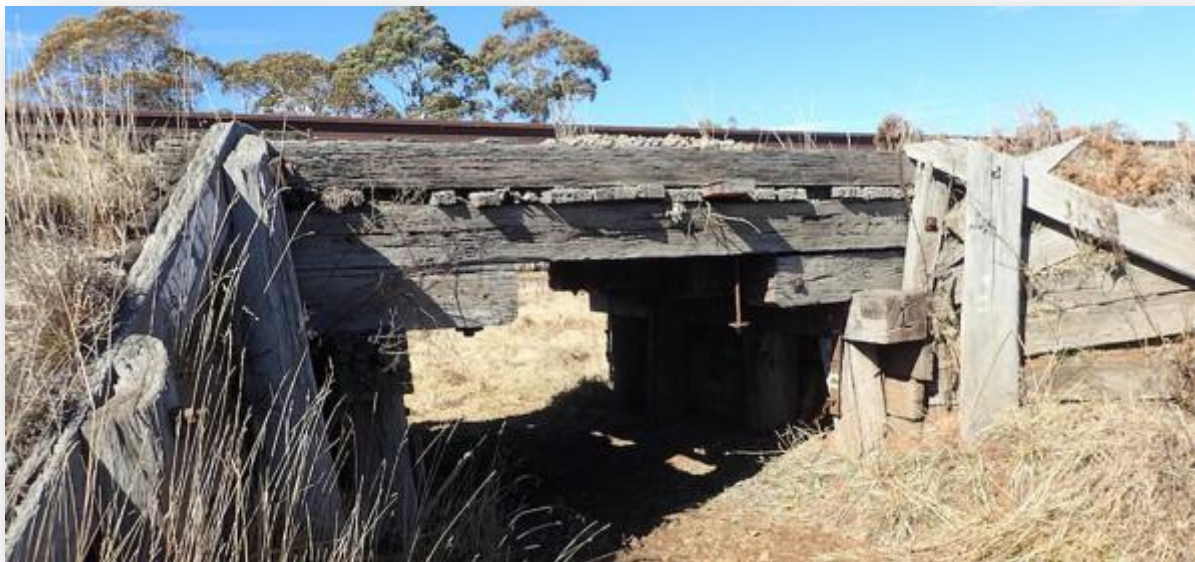
As with most railways, the corridor between Armidale and Glen Innes contains a number of old timber bridges. They will need to be re-furbished with users in mind, as well as for emergency and maintenance vehicles.
