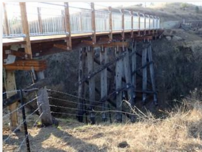
Above: Jimmy's Gully Bridge on the Brisbane Valley Rail Trail uses a combination of old (existing) and new timbers.
