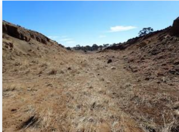
Side drains in some cuttings have completely disappeared with fill materials washed down from sides of cuttings.
