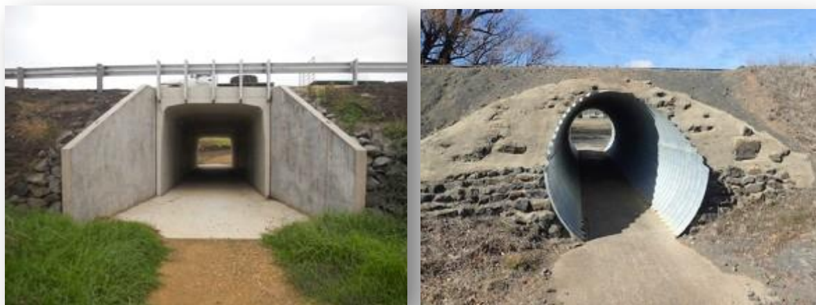
Underpasses at major roads are a solution to difficult road crossings. Above left: A concrete box culvert such as on the Port Fairy Warrnambool Rail Trail is one solution. Above right: A steel pipe has been put in the railway embankment at Guyra to provide pedestrian access from one side to the other.
