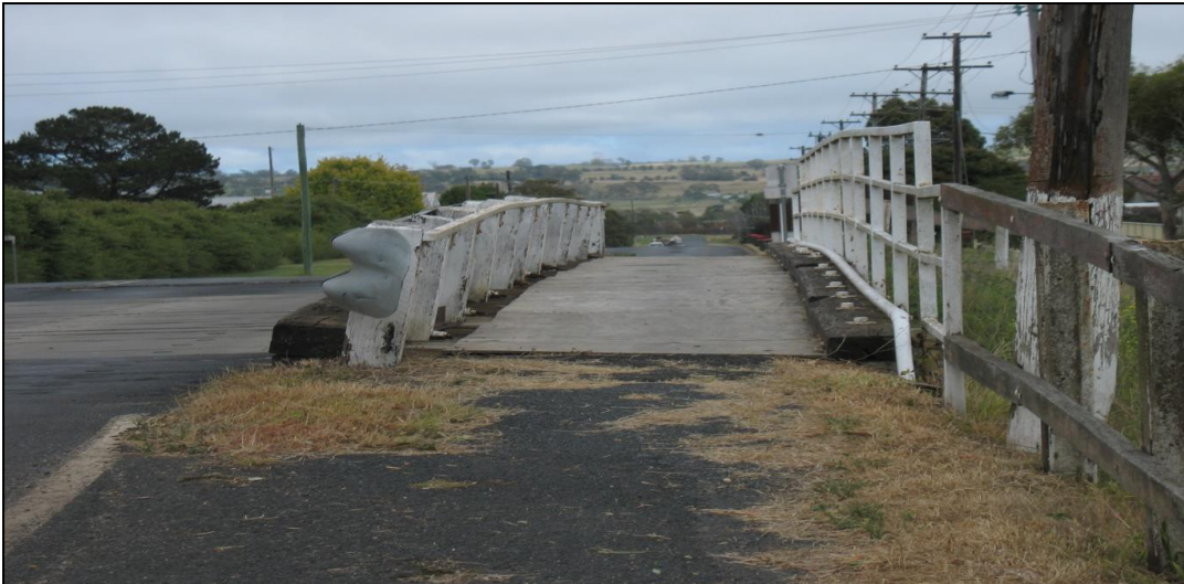
Lang Street Rail Overpass, Glen Innes
