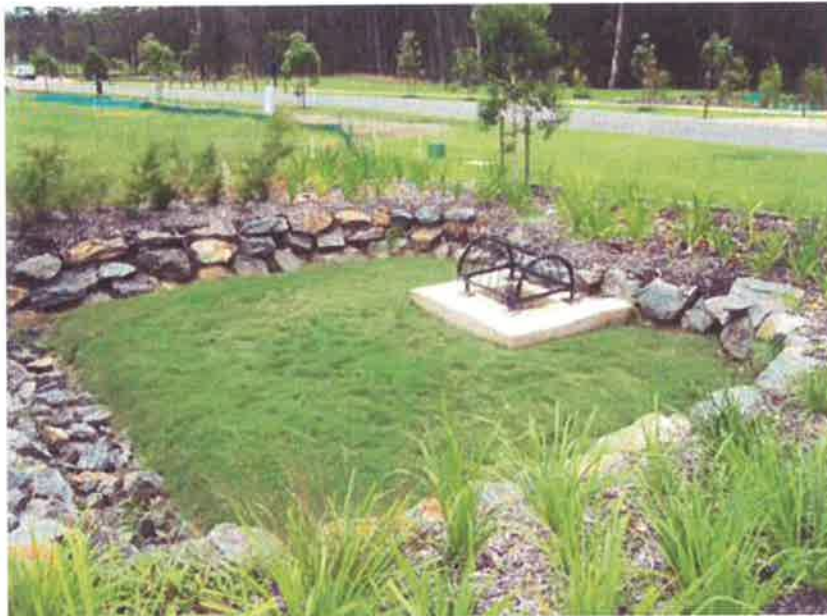
Figure 19: Culvert at end of under road drain and above riprap drain
