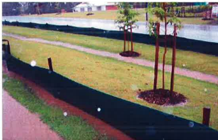
Figure 25: Filter fences and swale drain
