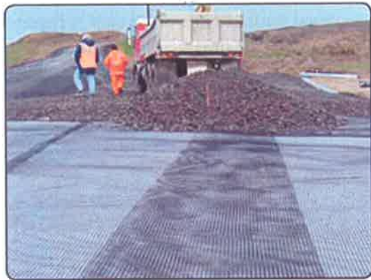
Tensar® grids create a stiffened raft
