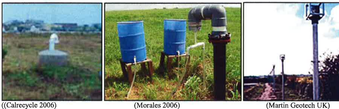
Figure 31: Head designs for passive vents
