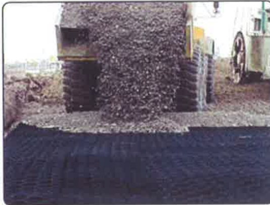
Ecocell® provides lateral support to fill material
