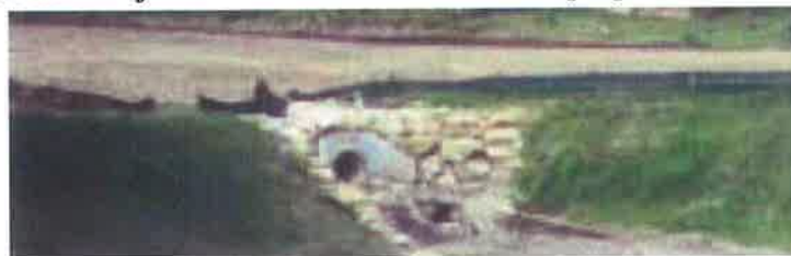
Figure 19: Culvert at end of under road drain and above riprap drain
