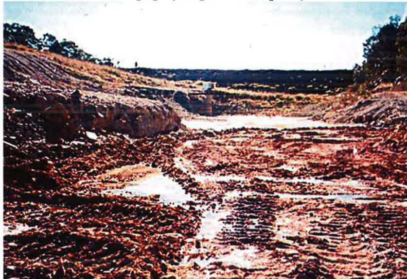
Photograph 4: Groundwater seepage (foreground) in quarry, June 2001
