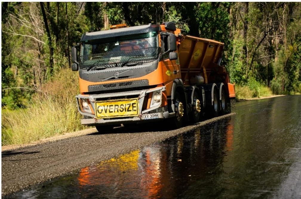
Image 1 – A graded aggregate bitumen seal being applied on Old Grafton Road
