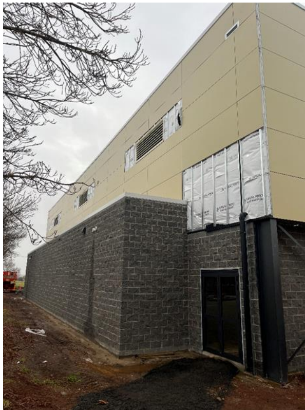
Image 1: Warwick Twigg Indoor Sport Stadium – progress on site
