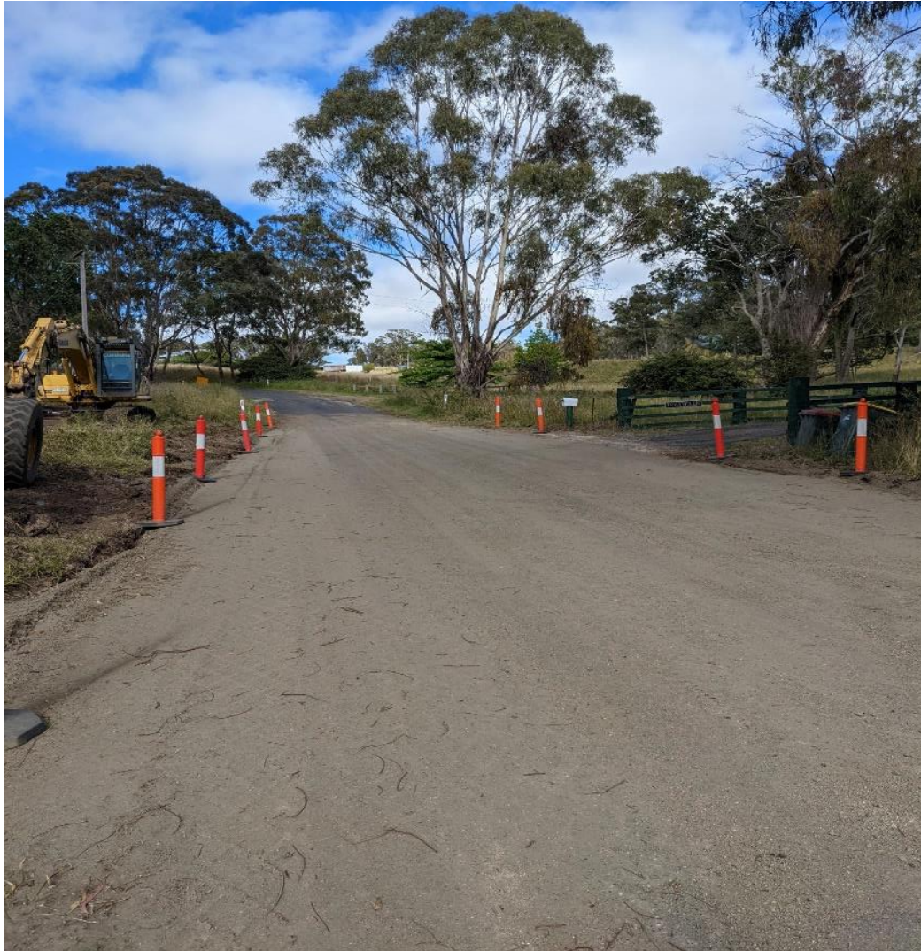
Image 3 – Blue Hills Road before seal has been applied
