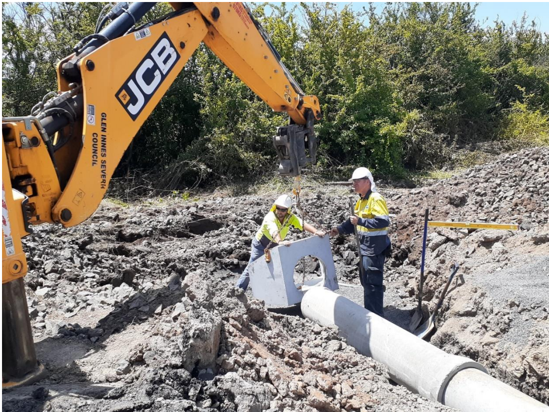
Image 2: Furracabad Road Rehabilitation – Work on-site
