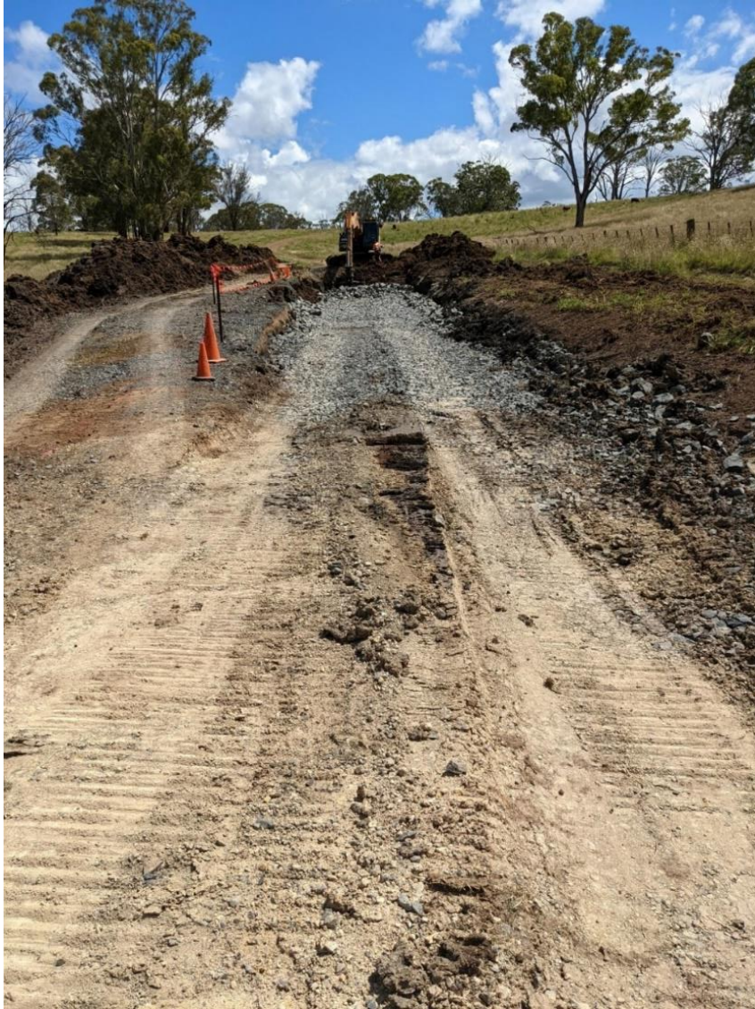
Image 4 – Ben Nevis Road subgrade being re-constructed
