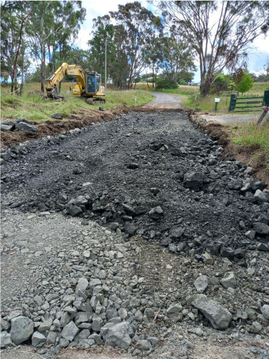
Image 2 – Blue Hills Road during construction
