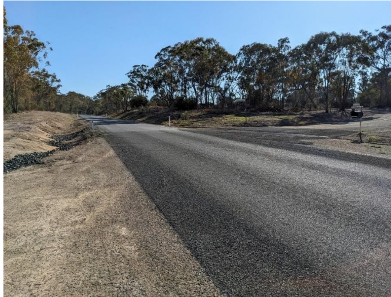
Image 7: Completed heavy patch on Wellington Vale Road.
