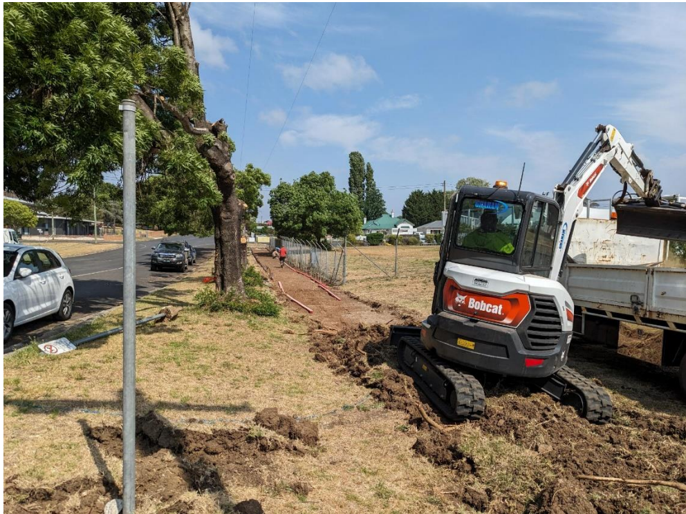
Image 3: Shared pathway construction
