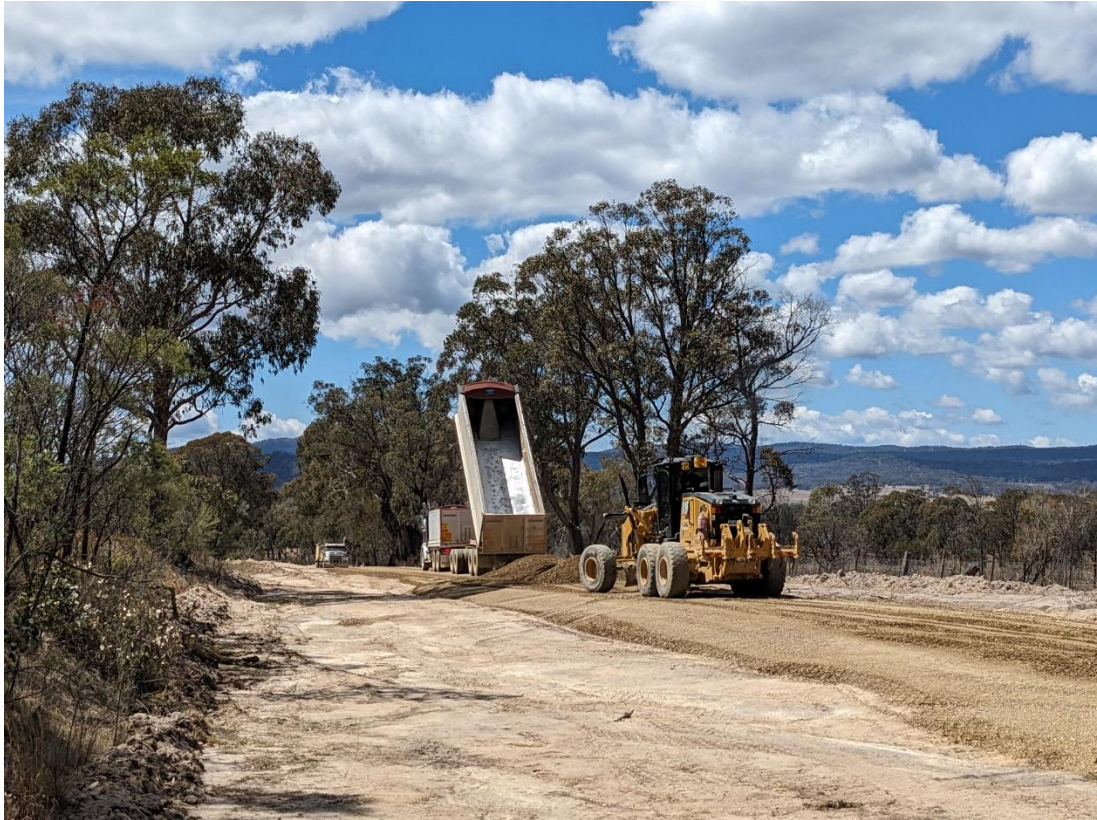
Image 2: Ten Mile Road gravel re-sheet
