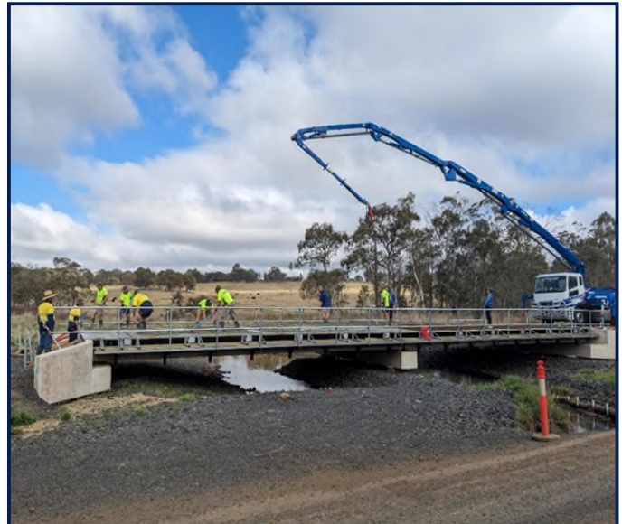
Bridge construction over Yarrow Creek on the Mt Mitchell Road
