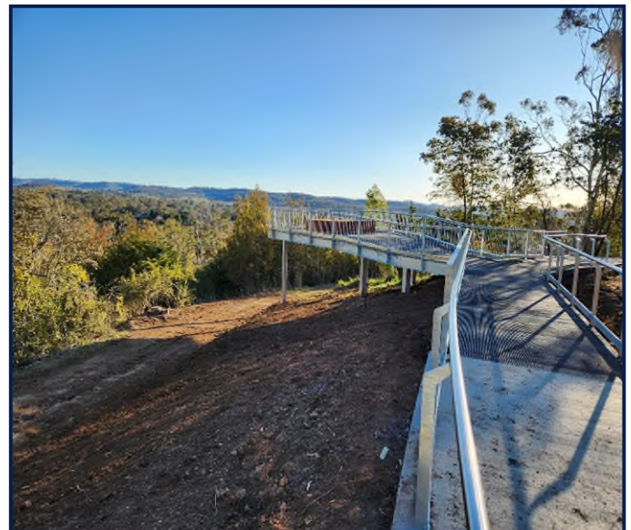
Skywalk under construction at Centennial Parklands
