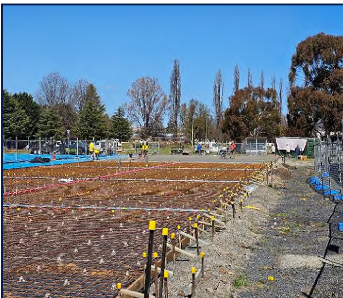
Outdoor courts under construction at Glen Innes Indoor Sports Centre
