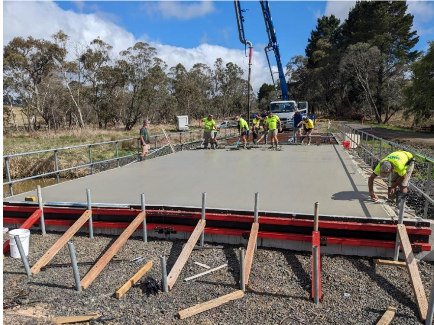
Image 2: Yarrow Creek bridge deck pour.
