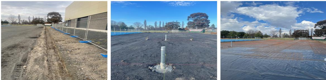
Images: Progress on the construction of the Outdoor Multi-Purpose Courts
