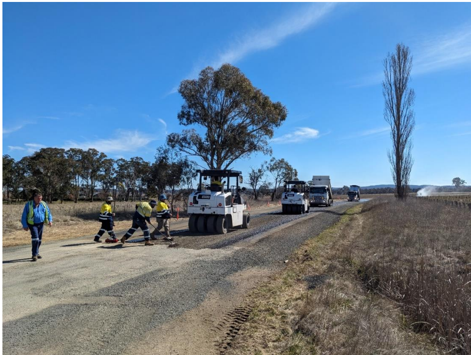
Image 4: Emmaville Road Segment 70
