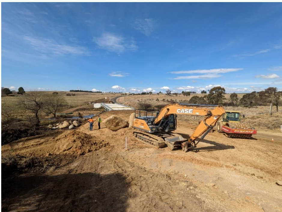
Image 2: Shannon Vale Bridge approach works
