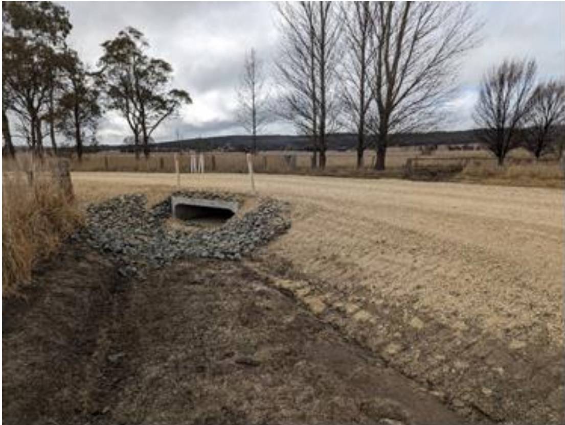
Image 2: Box culvert installation on West Furracabad Road
