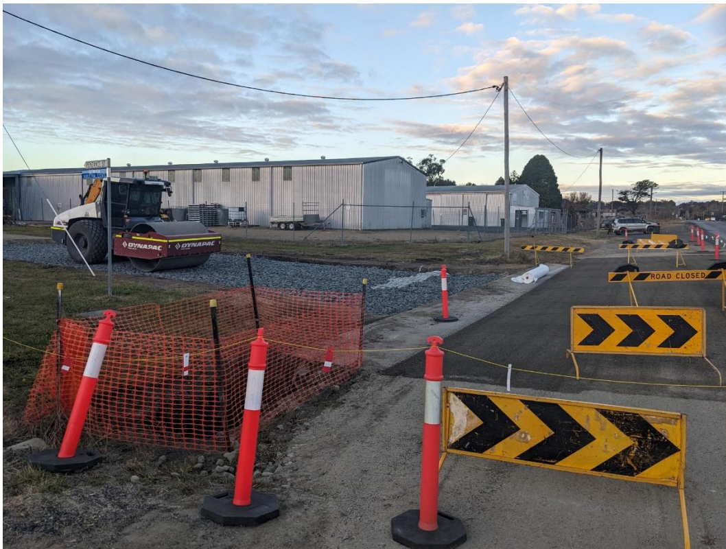
Image 4: Heavy patching on Grafton Street
