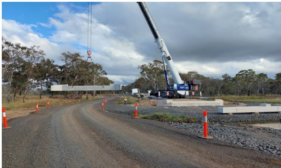
Image 1: Weir Built installing precast headstocks at Yarrow Creek Bridge
