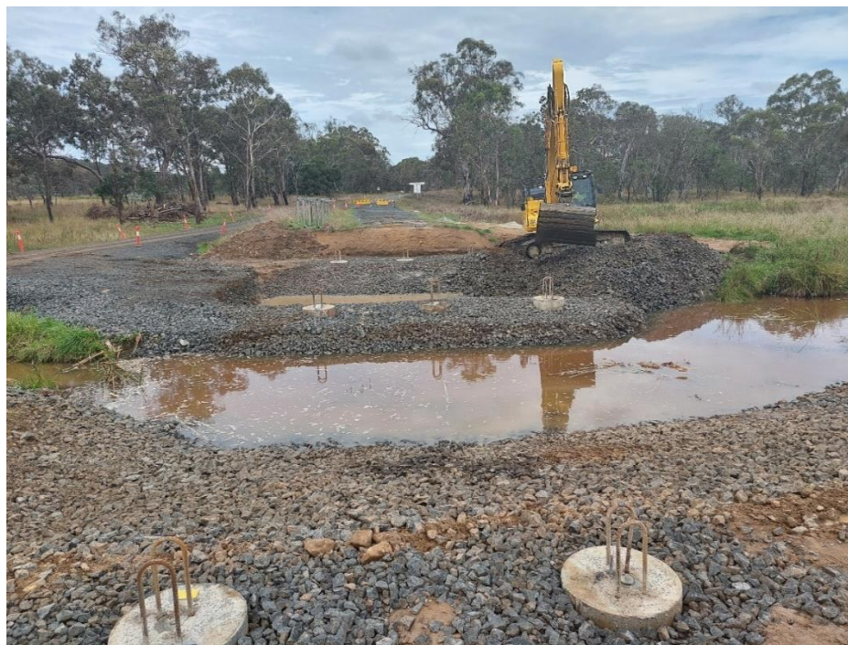
Image 1: Shaping scour protection on Yarrow Creek bridge foundations
