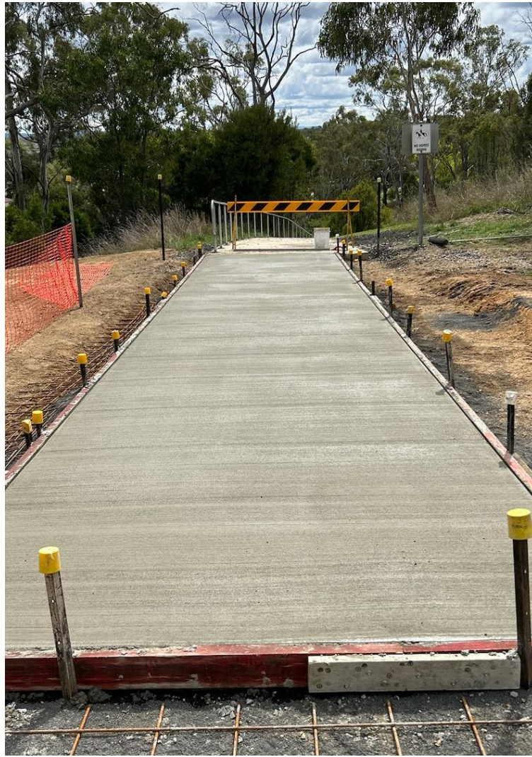
Image 3: Shared pathway construction on Tregurtha Way, Centennial Parklands
