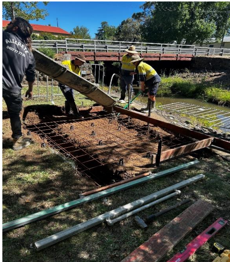
Image 2: Pedestrian bridge abutment construction on Wentworth Street
