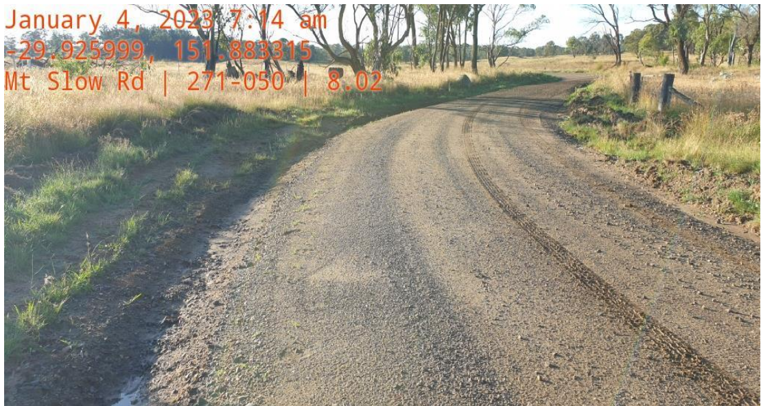
Image 5: A completed Mt Slow Road after gravel re-sheeting
