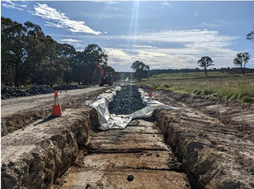
Figure 2: Rock Subgrade Replacement on Bald Nob Road - November 2022
