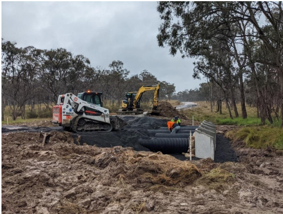
Image 4: Culvert replacement on Bald Nob Road.
