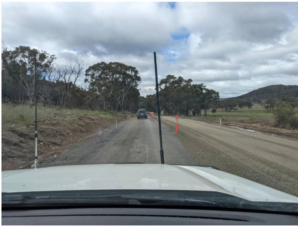
Image 2: Cement stabilisation of Emmaville Road segment 180
