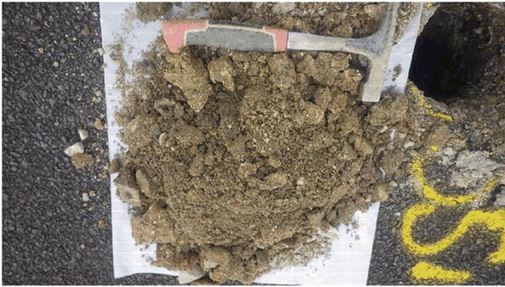
BH05 – Subgrade clay
