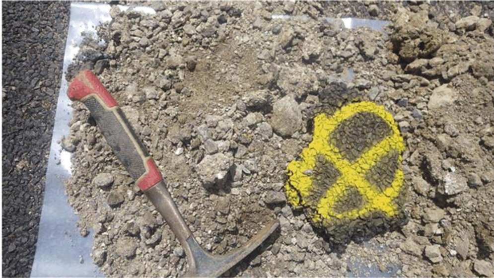
BH01 – Granular Base Course
