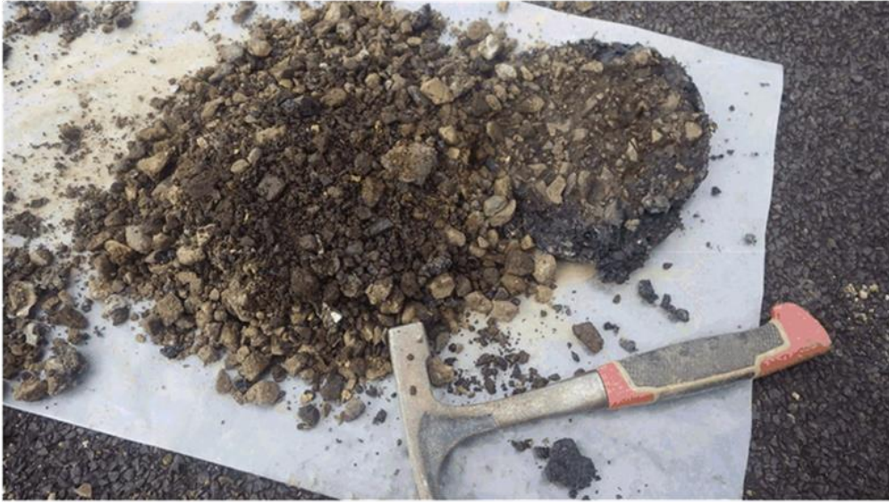
BH11 – Granular Base Course
