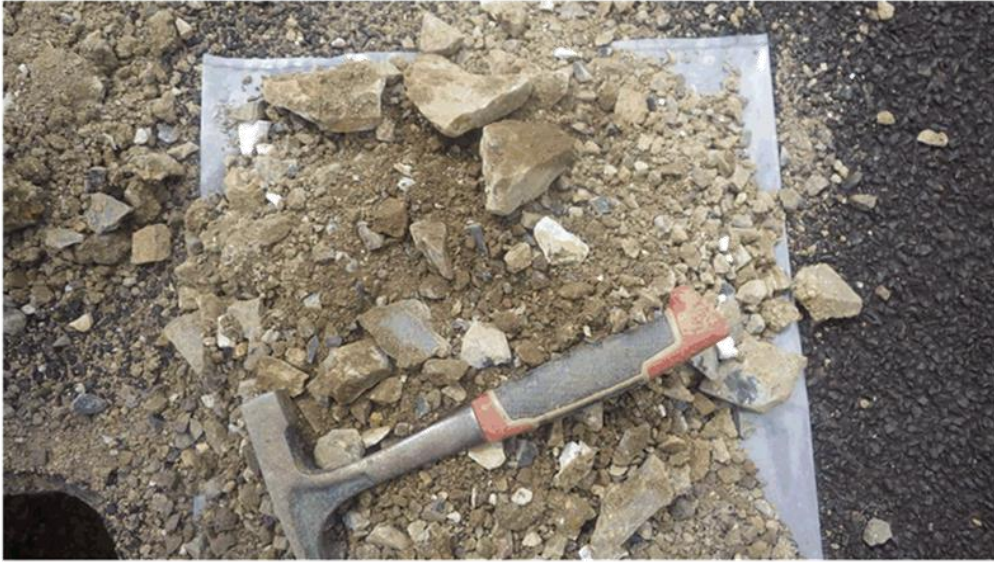
BH02 - Granular Subbase
