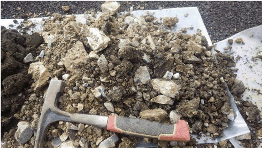
BH11 – Granular Subbase Layer
