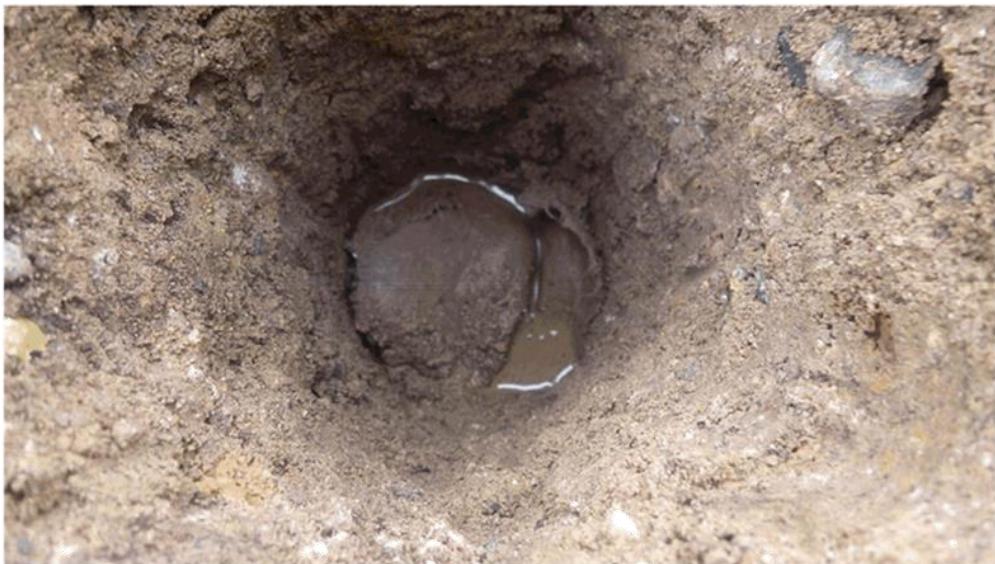
BH08 – BIDIM geofabric + free water at 390mm depth
