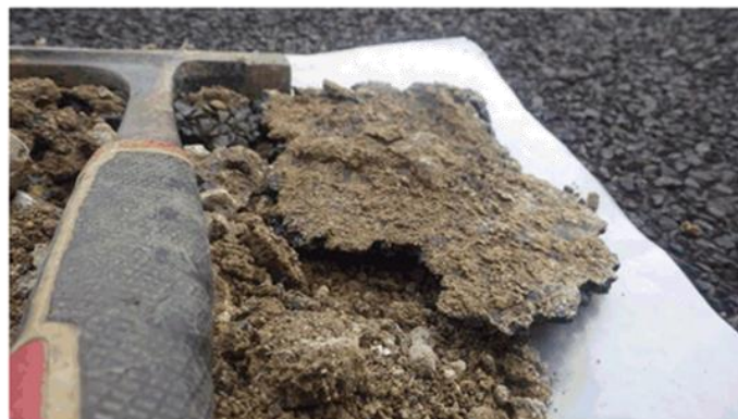
Figure 2 - Bitumen seal / granular interface poor adhesion
