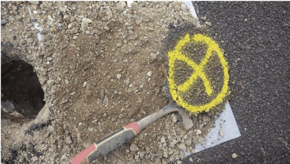
BH02 – Granular Base Course
