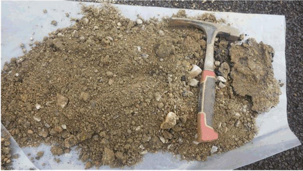
BH09 – Granular base course
