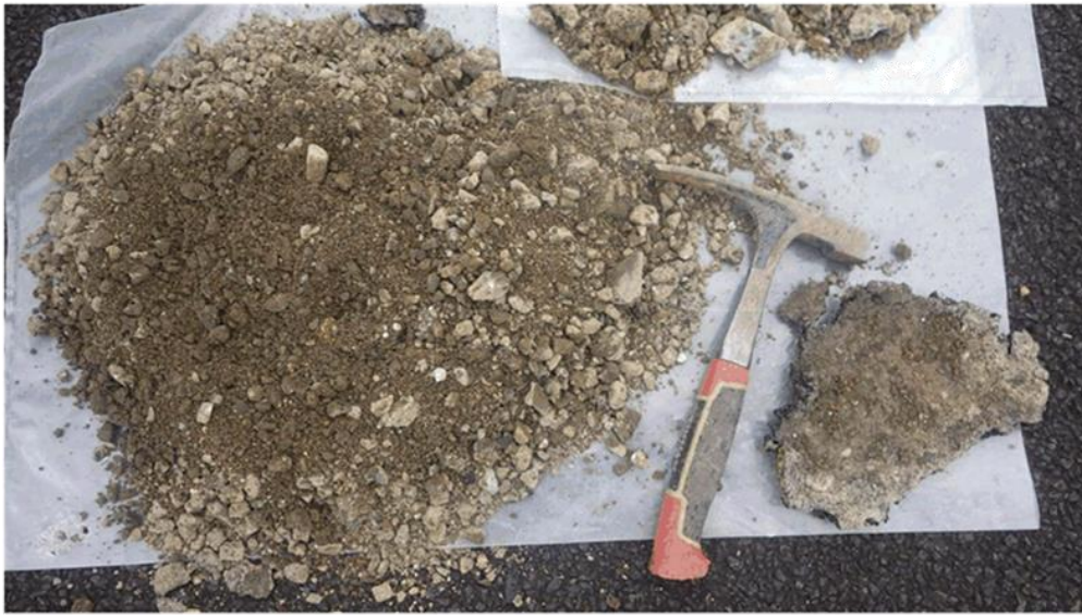
BH05 – Granular base layer
