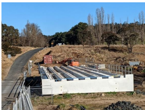
Image 2 – All pre-cast girders have been installed on the Shannon Vale Road bridge.
