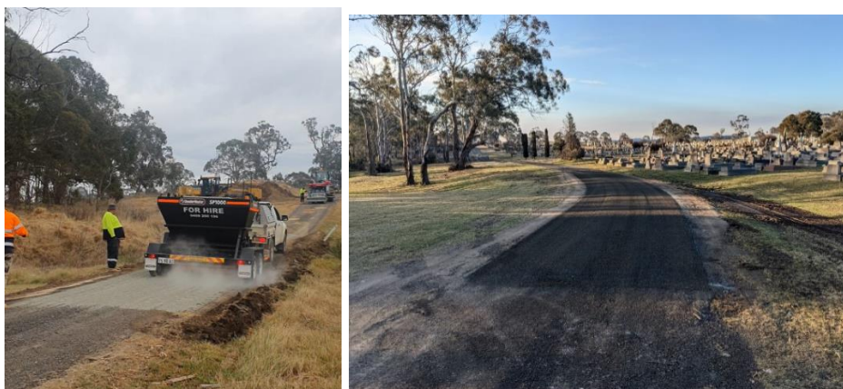
Image 1a and 1b – Pavement stabilisation trial with the Heavy Patch team at the Cemetery Loop Road
