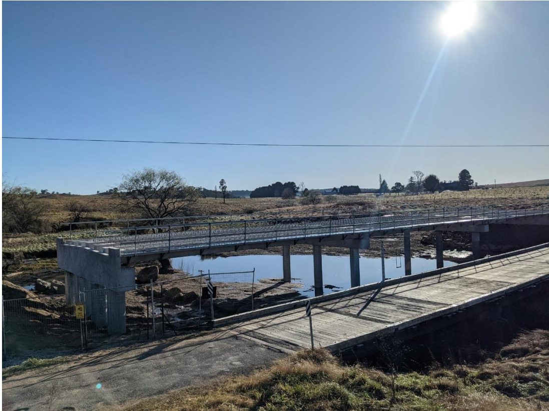
Image 3: Bridge girders installed over the Mann River on Shannon Vale Road.
