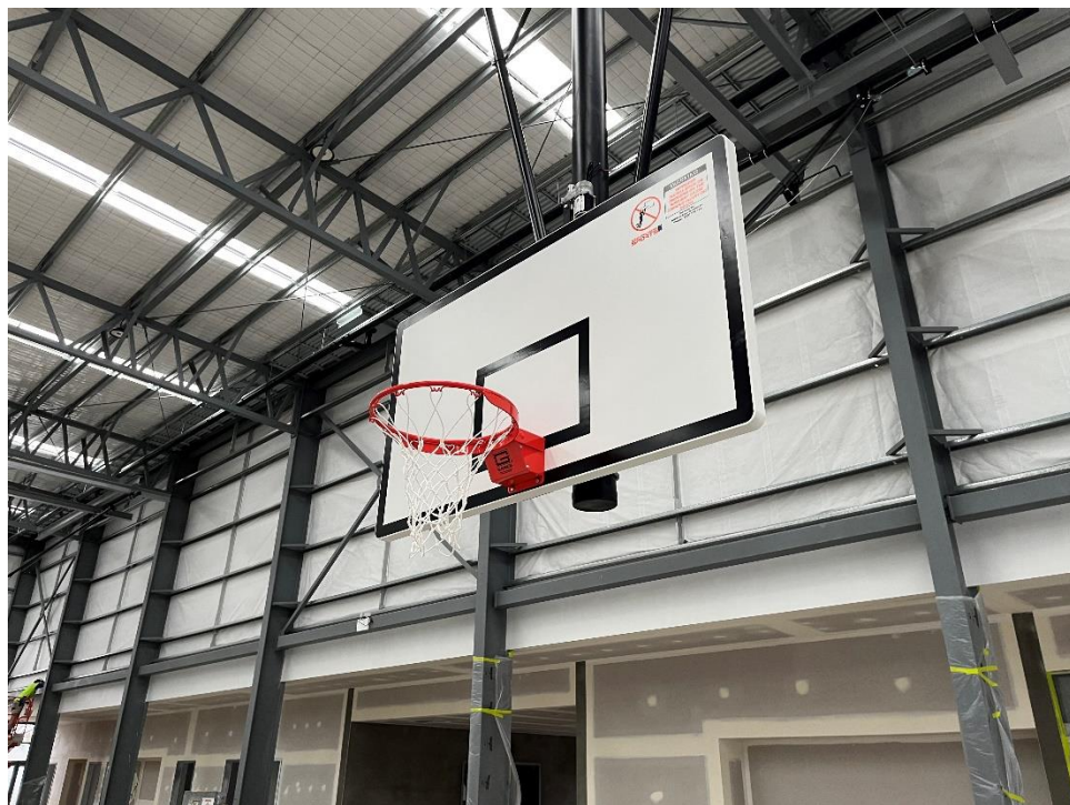
Image 1: Warwick Twigg Indoor Sport Stadium – progress on site
