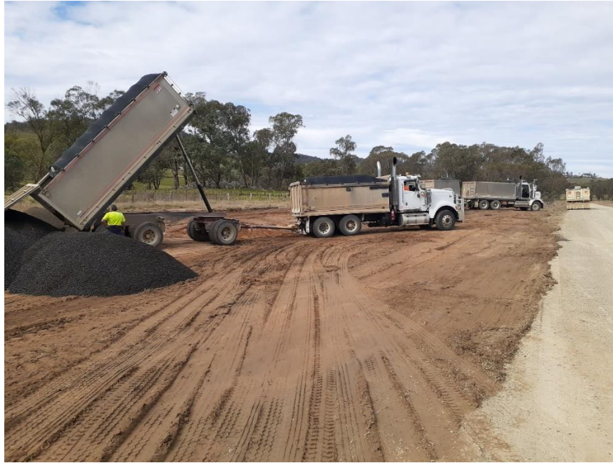
Image 2: Pinkett Road stockpile site
