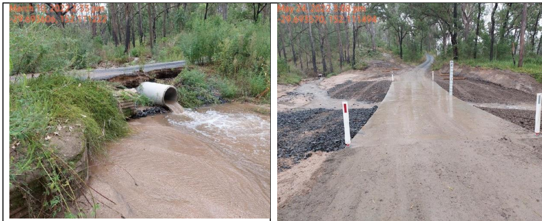
Image 1 – Completion of the new causeway on Stirrup Iron Creek Road
