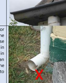
Stormwater should be piped or channelled away from the base of the building. Pooling of water at the base of the building can causes moisture in the foundations, rising damp in brickwork, attracts termites and can create more moisture in one part of the foundation than others leading to movement and cracking.
