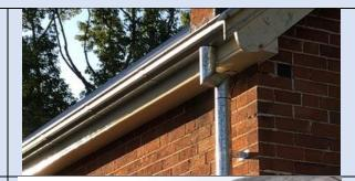
Low front quadrant profiled guttering
