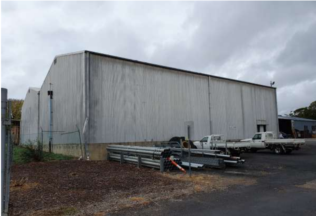
Figure 9: Western elevation of the subject building; the door to the right is to be replaced with a roller door
