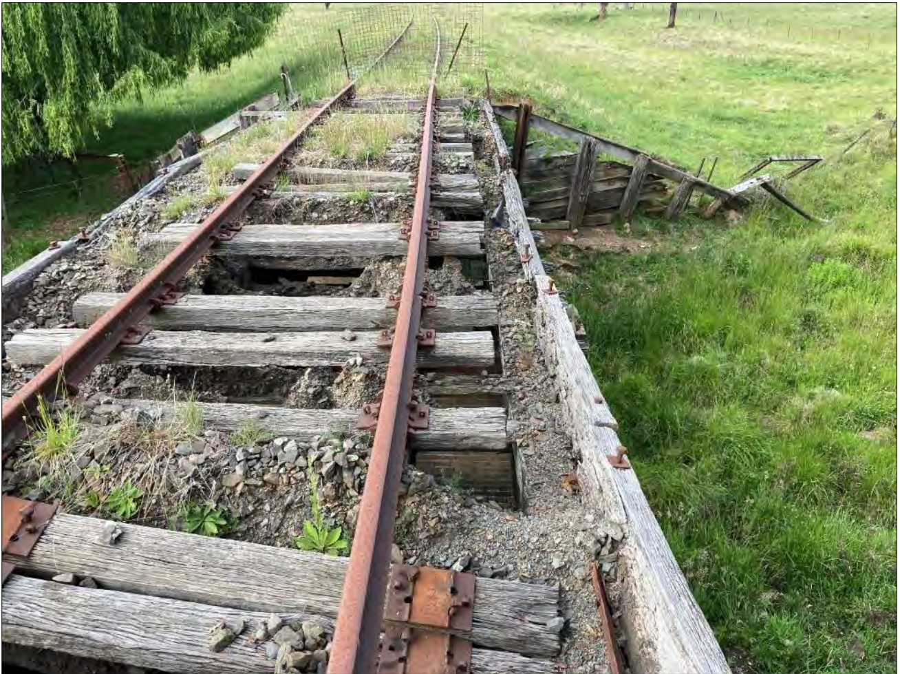
Figure 6-2: The deck planks that support the ballast rock are in very poor condition with many of the planks missing and large amounts of ballast have fallen out.
