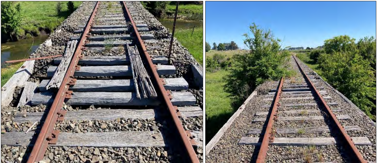
Figure 8-5: The timber transoms (rail ties) were found to be in a poor condition. If the bridge was to be repurposed for pedestrian and cycle use the timber transoms, railway line and rock ballast would be required to be removed. The existing timber edge rail that contains the ballast can left in place to act as a kerb/kick rail in the re-purposed bridge. To meet the current standards and Australian codes; vertical balustrade panels and a 1.4m high cycle rail will need to be installed. The current width of the bridge from inside of kerb to inside of kerb is approximately 3.0 metres which will result in a code compliant width for pedestrian bridges. As many of the deck planks are ‘falling’ out a new deck would be required for this bridge. The rock ballast can be reused to create the trail.
