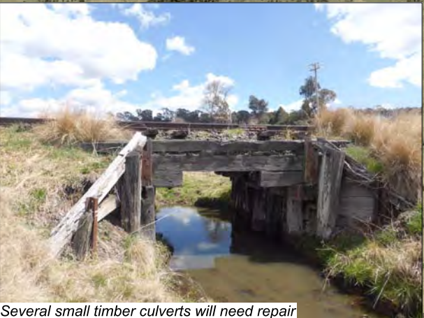
Several small timber culverts will need repair
