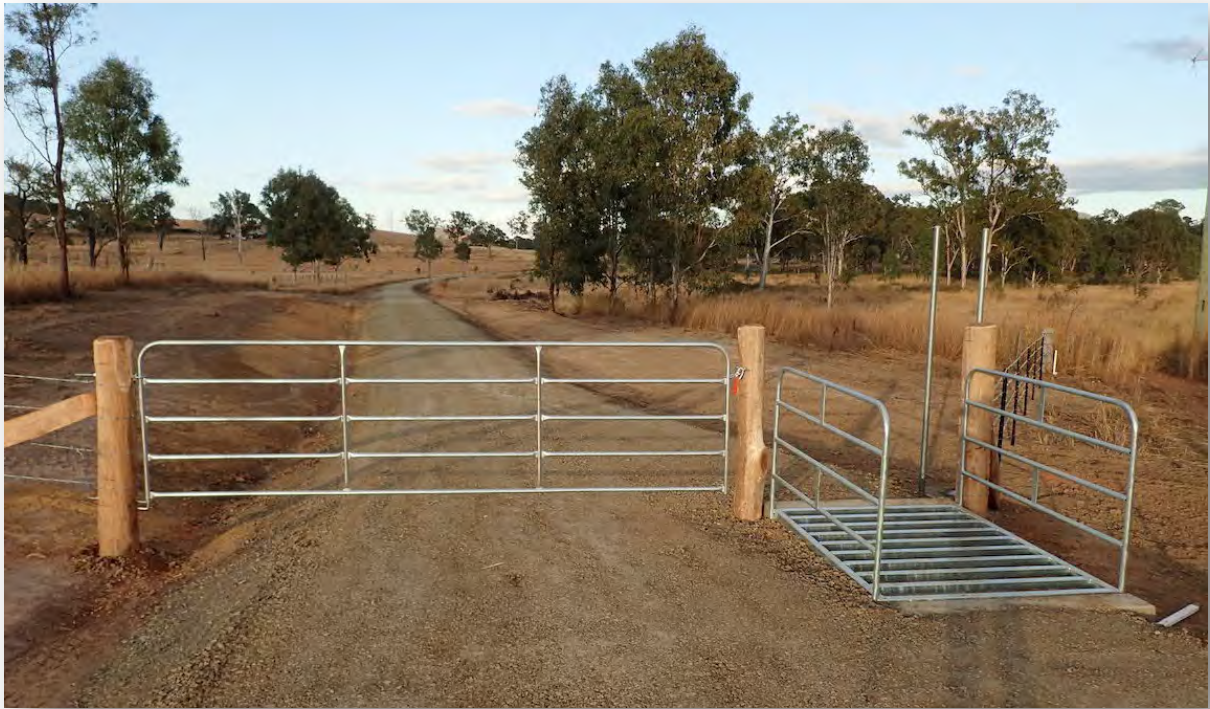
Above: a newly constructed management access gate and access grid on the Brisbane Valley Rail Trail (Qld).
