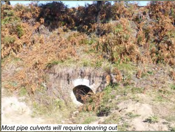
Most pipe culverts will require cleaning out
