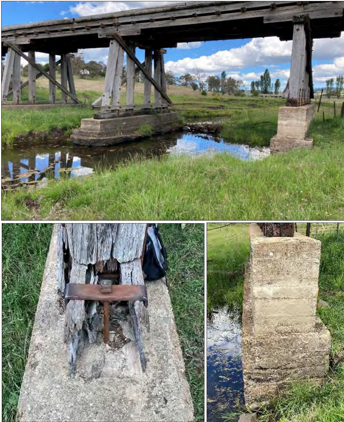
Figure 5-4: View of Spans 5 & 6 where the creek mainly flows. A close-up view of the decayed bottom cap that is vertically connected to and directly bearing on the concrete footing. Also the 2 concrete footing on either side of the main stream flow (Span 5) have signs of deterioration and scour. Scour protection (rip rap) is recommended to be installed.
