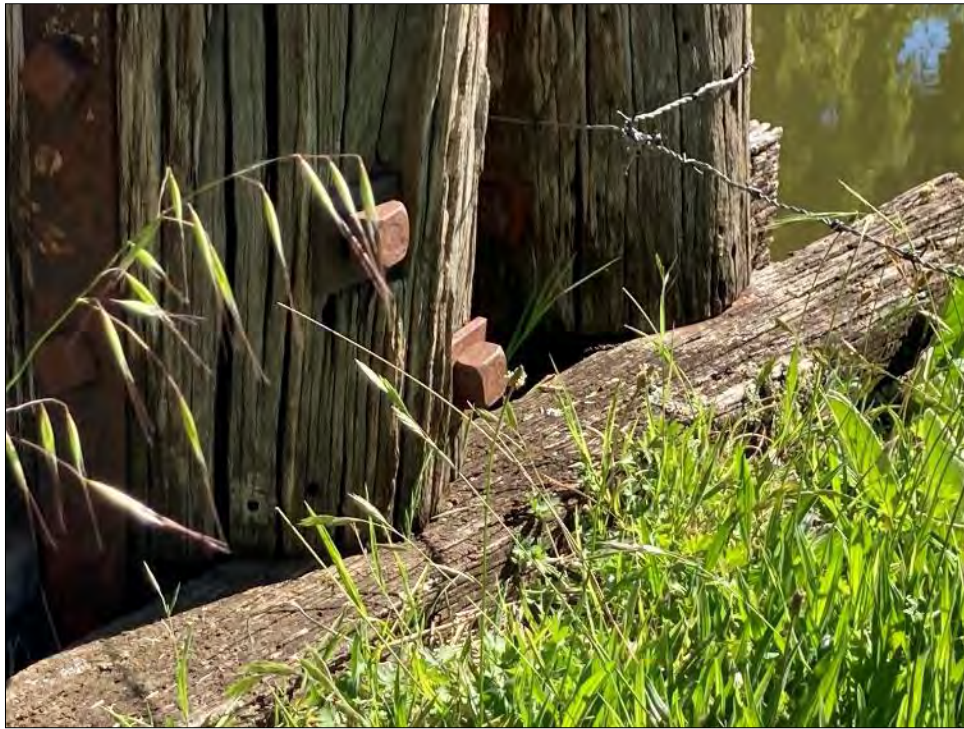
Figure 8-3: It was noted that the bottom section of several posts and timber cap wales have started to undergo decay. This is as expected due to the timber posts bearing directly on the concrete footing which typically has a high moisture content. Over time the timber post undergoes capillary action and draws up the moisture like a ‘straw’. Once the moisture content in the timber elements reaches 22%, decay causing fungi are activated and the decay process begins. Overall the timber bents were found to be in poor condition. The bottom sections of the timber piles were determined to be a ‘hotspot’ for decay and determined to be an ideal area to test using non-destructive methods, such as EPHOD® Stress Wave Technology. Refer to Appendix B for more information of this type of testing method. A reading of above 1500 \mu s was recorded for the time taken for the compression wave to travel across the section of the member tested. This was recorded at the bottom of one of the piles (left image above) and was found to be similar across most of the piles/posts. Deterioration of this magnitude means that the Modulus of Elasticity/Modulus of Rupture in various stress directions (wood is anisotropic with different strength properties in different directions) has deteriorated to an extent that the element can no longer support its own dead weight. Readings between 1000 \mu s and 2200 \mu s indicate that the member cannot carry its own dead weight in these regions. Readings in excess of 2200 \mu s can signify a cavity while a reading above 3300 \mu s indicates the element can no longer support its own dead load and is at risk of failing at any point.
