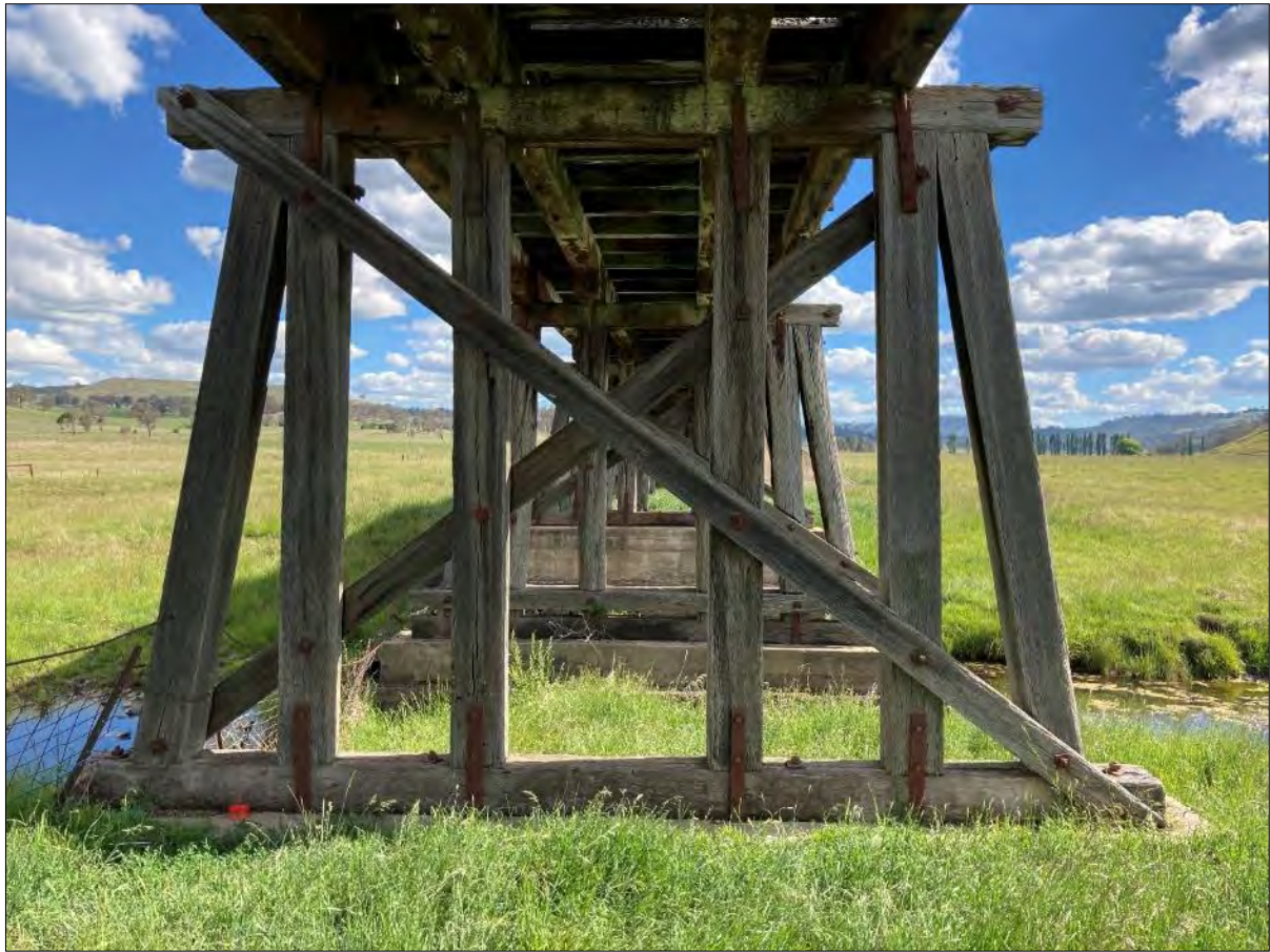
Figure 5-3: View of the typical timber pile bent configuration. The bent comprises of 6 square (or round) dimensional post bearing directly on a timber bottom cap which is vertically connected to the concrete footing. The bent is also supported by cross bracing that provides adequate support for the 2.5-4m long posts. Overall the timber bents were found to be in a poor condition with the timber bottom caps being in the worst condition. This is as per expected due to the timber bearing directly on the concrete footing which typically has a high moisture content. Over time the timber post undergoes capillary action and draws up the moisture like a ‘straw’. Once the moisture content in the timber elements reaches 22%, decay causing fungi are activated and the decay process begins. This timber bottom cap has partially ‘protected’ the timber posts which are in relatively poor condition, however the timber cap wales will cost a significant amount to be replaced or repaired in-situ.
