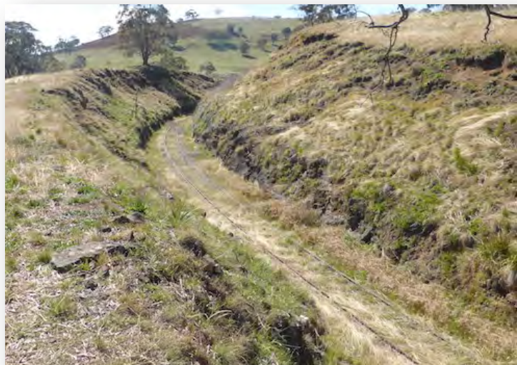
The old drains of the many cuttings along the proposed rail trail will require attention to ensure they still perform the task of clearing water from the cuttings.
