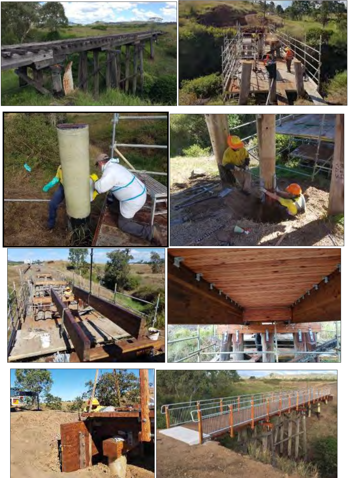
Figure 11-4: The photo series above demonstrates Option 2 type of fix that was done for Jimmy Gully Bridge along the BVRT. The existing poor condition superstructure was removed and the piles were repaired with high strength fibre or posted with new section. New glulam back wall, caps, girders and deck system was installed utilising a horizontal connection detail.
