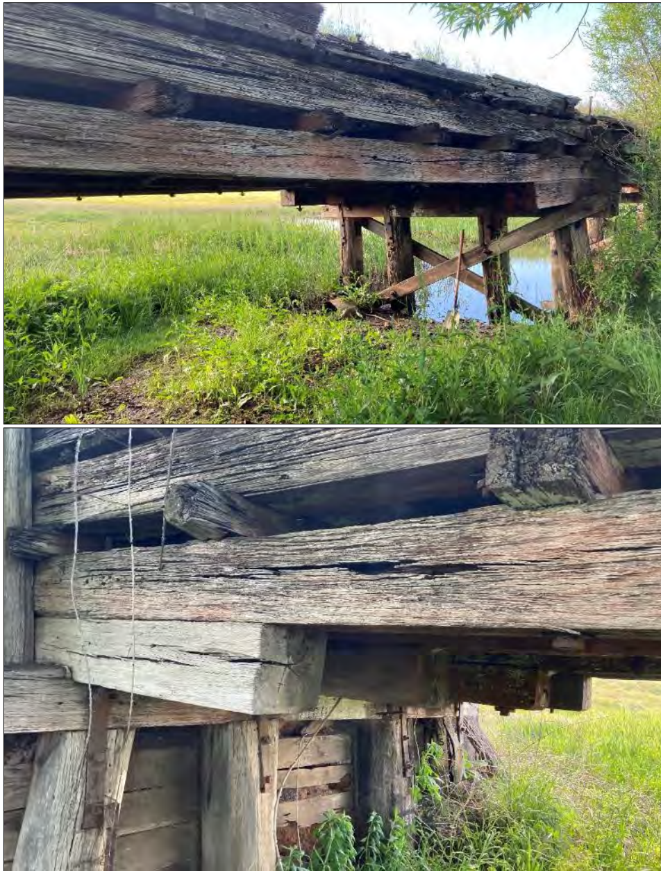
Figure 7-2: The superstructure and deck are the same configuration and similar condition as Manrowan Creek Bridge. The girders are in very poor condition with Girder 4 in Span 1 having visible cavities and excessively deflecting under its own deadload which has result in full length cracking.
