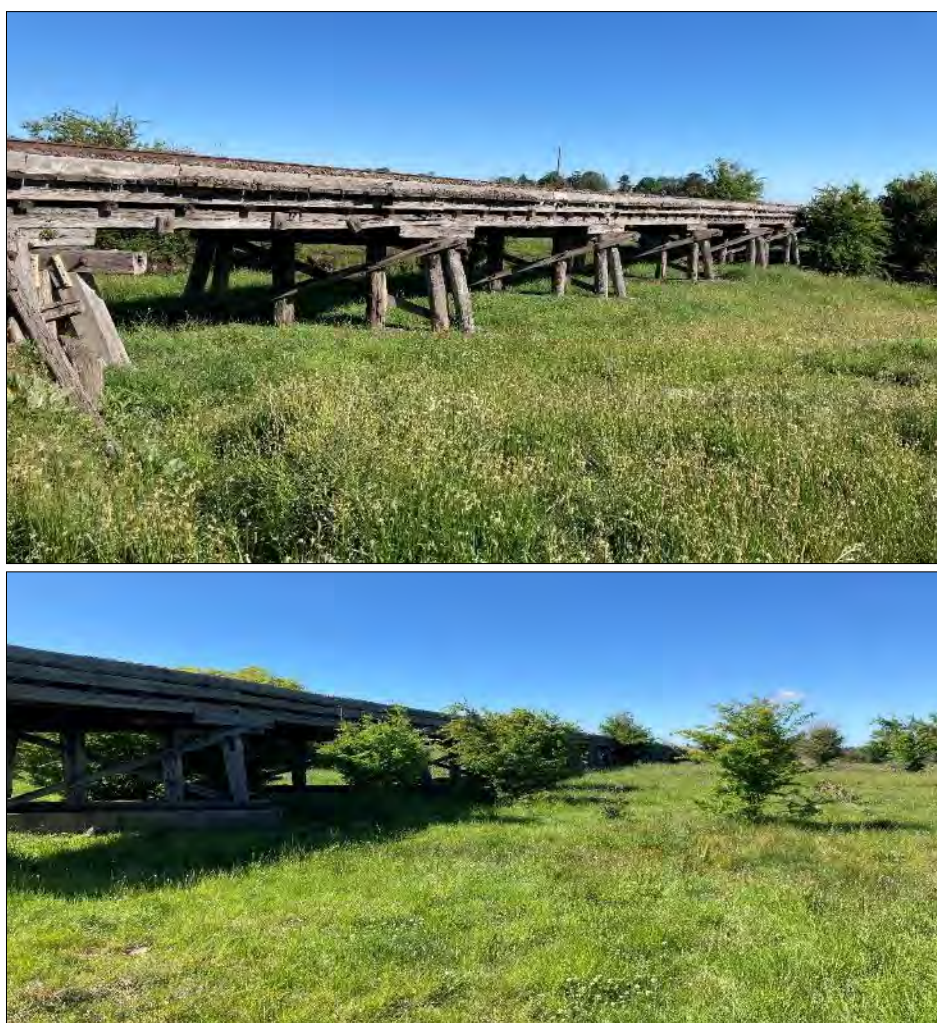
Figure 8-1: Top image is the view of Beardy Waters Bridge from Abutment 1 and the bottom image is from Abutment 2. The timber bridge is 14 spans long and approximately 112 metres in length (8 metre long spans). Note several of the spans at Abutment 2 side of the river are in very poor (unsafe) condition and have partially collapsed and sunken.
