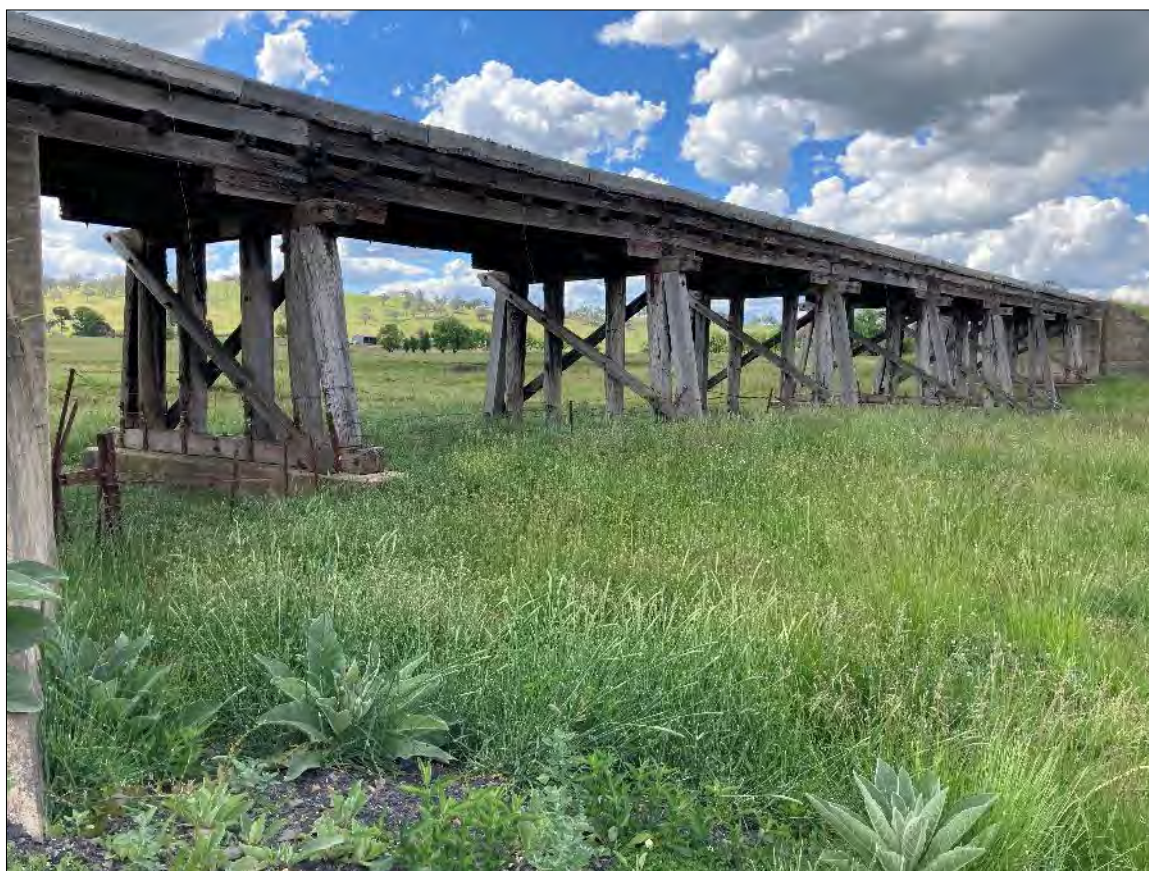
Figure 5-1: View of Manrowan Creek Bridge from the Abutment 1 end of the structure. The timber girder under bridge has 8 spans in total with an overall length of 56m. This type of design was quite common for the longer spans that transverse over the larger creeks along the New England Railway line. At the time of inspection there no water flowing in Manrowan Creek, only a pool of water approximately 1m deep at spans 5 & 6.
