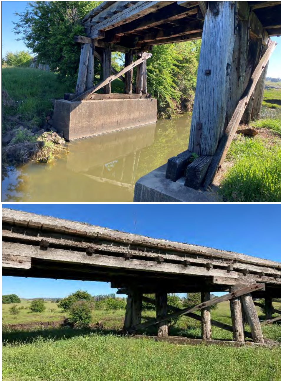
Figure 8-2: View of the typical timber pile bent configuration. The bent comprises of 6 square (or round) dimensional post bearing directly on a timber bottom cap which is vertically connected to the concrete footing. The bent is also supported by cross bracing that provides adequately support for the 2.5-4m long posts. Overall the timber bents were found to be in a poor to very poor condition with the timber bottom caps being in the worst condition. This is as per expected due to the timber bearing directly on the concrete footing which typically has a high moisture content. Over time the timber post undergoes capillary action and draws up the moisture like a ‘straw’. Once the moisture content in the timber elements reaches 22%, decay causing fungi are activated and the decay process begins. This timber bottom cap has partially ‘protected’ the timber posts which are in relatively poor condition, however the timber cap wales will cost a significant amount to be replaced or repaired in-situ. Also note the bents are heavily skewed (approximately 30 degrees) and are parallel with the stream.
