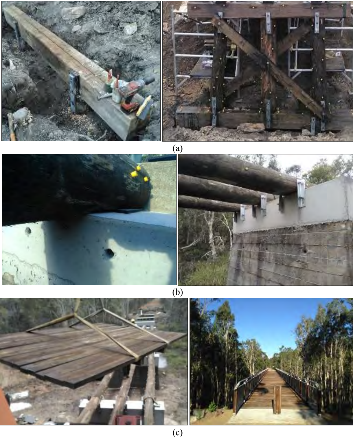
Figure 11-3: The above photo series demonstrates Option 1 type of fix (hardwood) used for the construction of two Mary to Bay Rail Trail Bridges. Seen above in photo (a) is the construction of a frame bent using an intermediate cap which was installed on top of the existing pile stubs. This allowed the hardwood posts, cross bracing and cap to be installed at the correct reference height. Also note the yellow plugs that indicate that Decaystop® rods have been installed. Photo (b) shows the girders being installed using a horizontal connection system and a rubber liner between the timber girder and concrete pier. In photo (c) the pre-panelised deck is installed along with the modulus handrail and cycle rail system.
