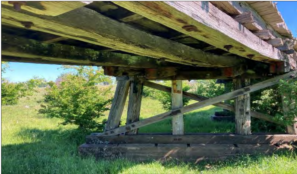
Figure 8-7: A view of a section of the bridge that has collapsed/sunken at Span 11. These members will require replacement before the bridge can be reopened for pedestrian and cycle use. The superstructure comprises of 4 girder lines per span with the 2 girders per a girder line (8 girders per span in total). The double stacked girders are separated by traverse beams that contribute to the load sharing ability of the superstructure.
