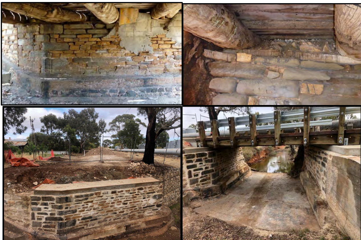
Figure 11-6: The brick abutments and the hardwood deck and girders at Shannon Road Bridge were in very poor condition with major refurbishments required. The abutment wall was repaired where the mortar was missing due to weathering and scour. The abutment wall was levelled off in preparation for a loadbearing sill pad for the girders. Once the abutments were repaired a new hardwood girder and deck system was lifted into position and the bridge now has a load rating of 15 Tonne.
