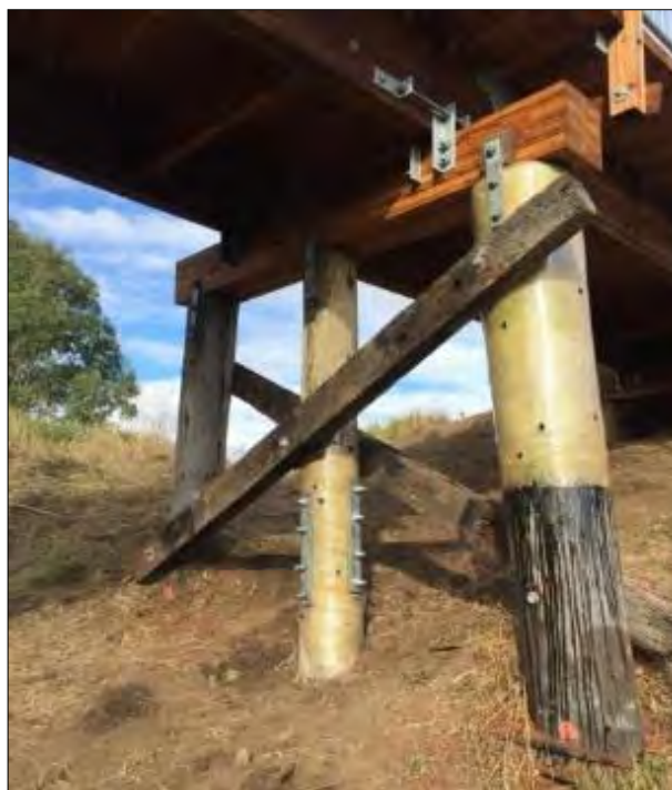
Figure 11-9: Diffuser (Borate Salt) rods are installed in the remaining hardwood elements in order to resist further deterioration of the timber caused by fungi growth. Note the red bungs are the decay ‘hotspots’ where the timber is prone to have a higher moisture content. These holes are required to be checked for rod depletion as per the issued maintenance manual (typically every 2-5 years depending on environmental conditions).
