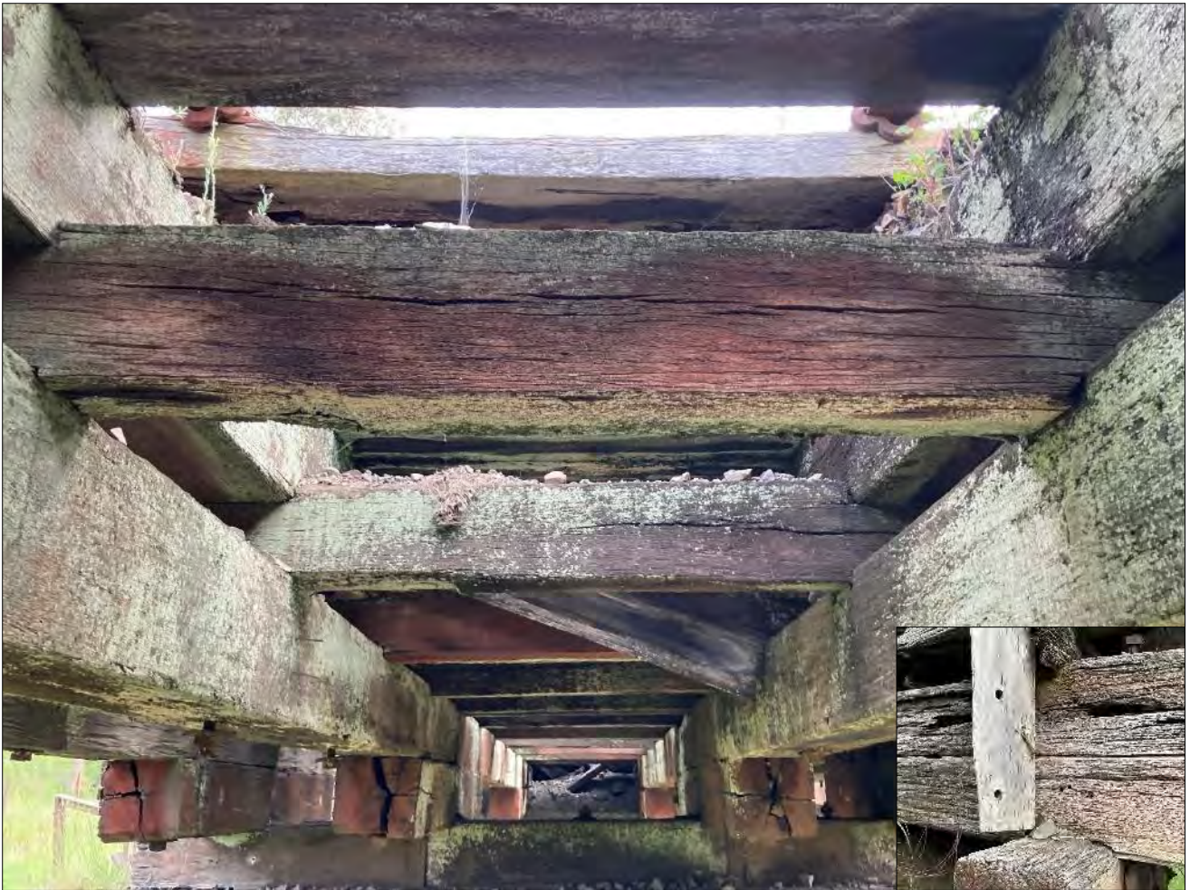
Figure 6-5: A view of the underneath section of the bridge. It can be seen that the deck has collapsed in sections along the bridge. These planks will require replacement before the bridge can be reopened for pedestrian and cycle use. The superstructure comprises of 4 girder lines per span with the 2 girders per a girder line (8 girders per span in total). The double stacked sawn square girders are separated by traverse beams that contribute to the load sharing ability of the superstructure. Several of the girders has undergone significant deterioration with large splits visible from the underneath. The girders and corbels are connected with large vertical through bolts. Vertical fasteners increase the rate of decay in timber as they allow moisture to travel down the fastener into the heartwood of the girders and corbels where evaporation is more difficult, therefore increasing the moisture content in the middle of these elements over longer periods of time. The heartwood of a large dimensional element is less capable of breathing and expelling moisture than the sapwood that surrounds it, so vertical connectors funnel the moisture directly into the heartwood accelerating decay. Once the moisture content exceeds 22%, timber consuming fungi are activated and the decay process begins. Refer to Figure 3-2 for a detailed description of how and where the decay occurs due to these vertical bolts.
