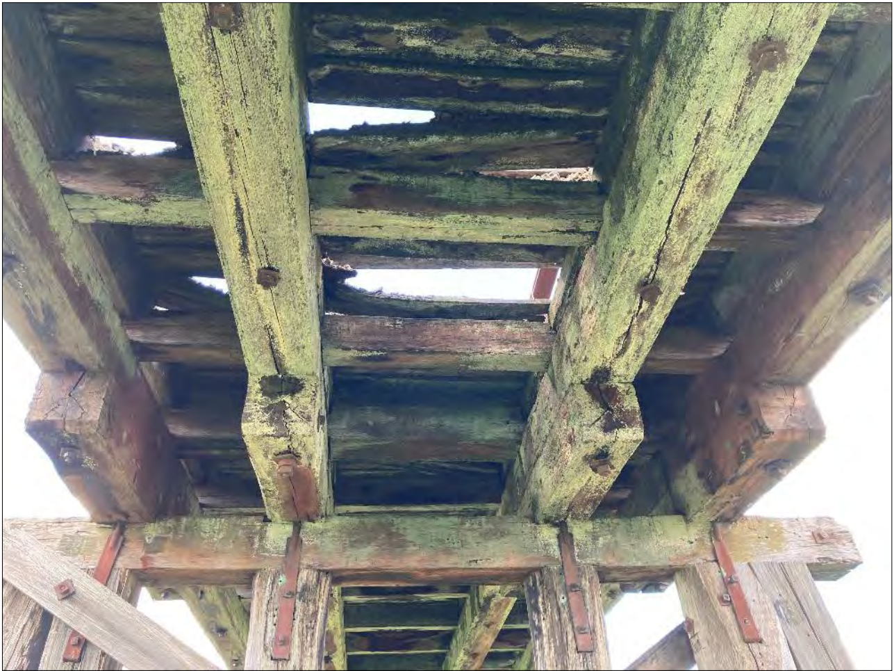
Figure 5-2: A view of the underneath section of the bridge. It can be seen that the deck has collapsed in sections along the bridge. These planks will require replacement before the bridge can be reopened for pedestrian and cycle use. The superstructure comprises of 4 solid sawn girder lines per span with the 2 girders per a girder line (8 girders per span in total). The double stacked girders are separated by traverse beams that contribute to the load sharing ability of the superstructure. Generally the transverse beams were in poor condition and the girders are in poor-very poor condition. One of the girders has undergone significant deterioration with large splits visible from the underneath as well as being covered fully in decay fungi growth. The girders and corbels are connected with large vertical through bolts. Vertical fasteners increase the rate of decay in timber as they allow moisture to travel down the fastener into the heartwood of the girders and corbels where evaporation is more difficult, therefore increasing the moisture content in the middle of these elements over longer periods of time. The heartwood of a large dimensional element is less capable of breathing and expelling moisture than the sapwood that surrounds it, so vertical connectors funnel the moisture directly into the heartwood accelerating decay. Once the moisture content exceeds 22%, timber consuming fungi are activated and the decay process begins. Refer to Figure 3-2 for a detailed description of how and where the decay occurs due to these vertical bolts.
