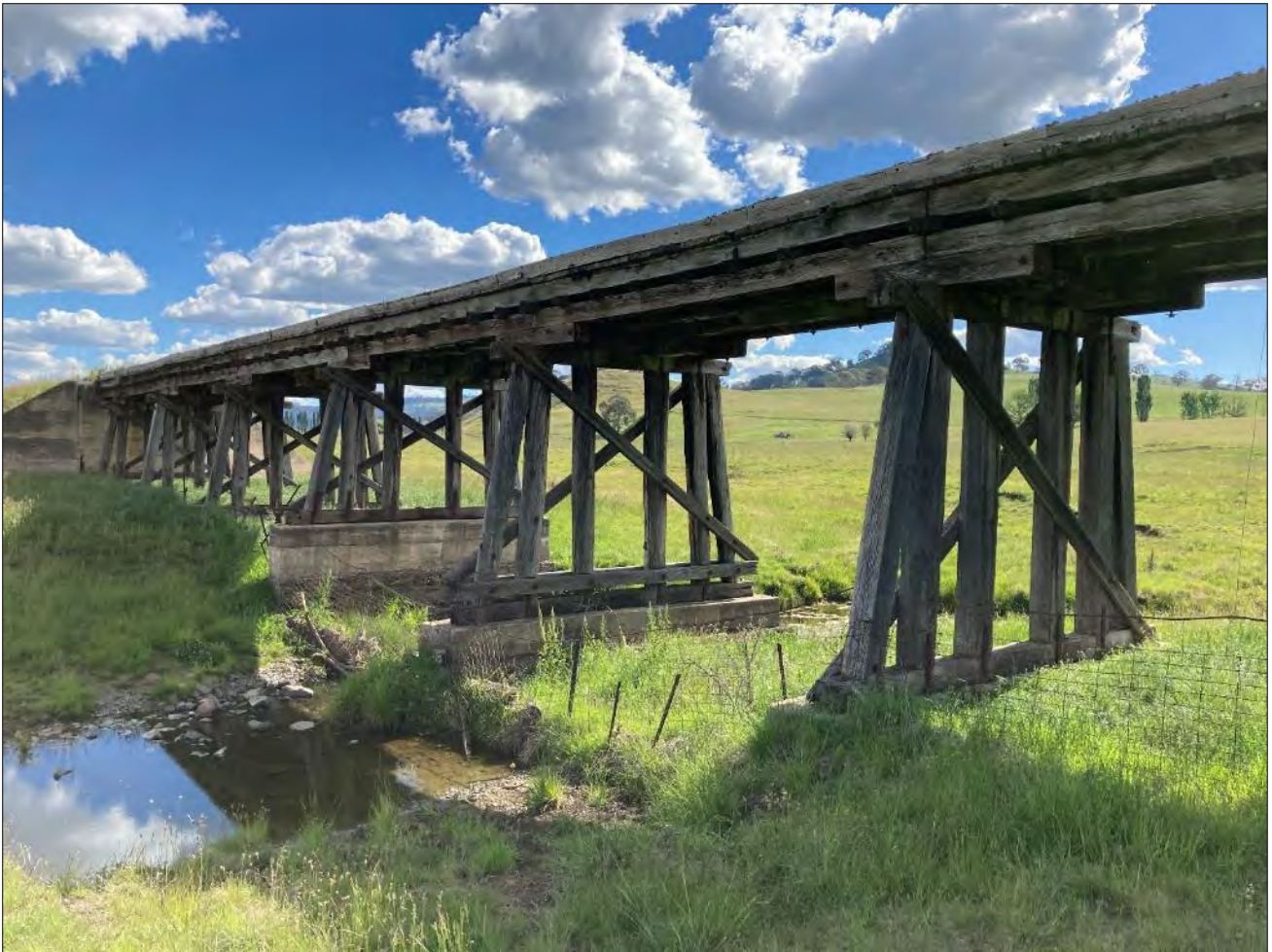
Figure 5-10: View of Manrowan Creek from Abutment 2 side of the creek. Note the fence attached to the bridge which can have a negative impact on the bridge due to the increased chance of debris getting trapped and thus the lateral loads on the bridge increase.
