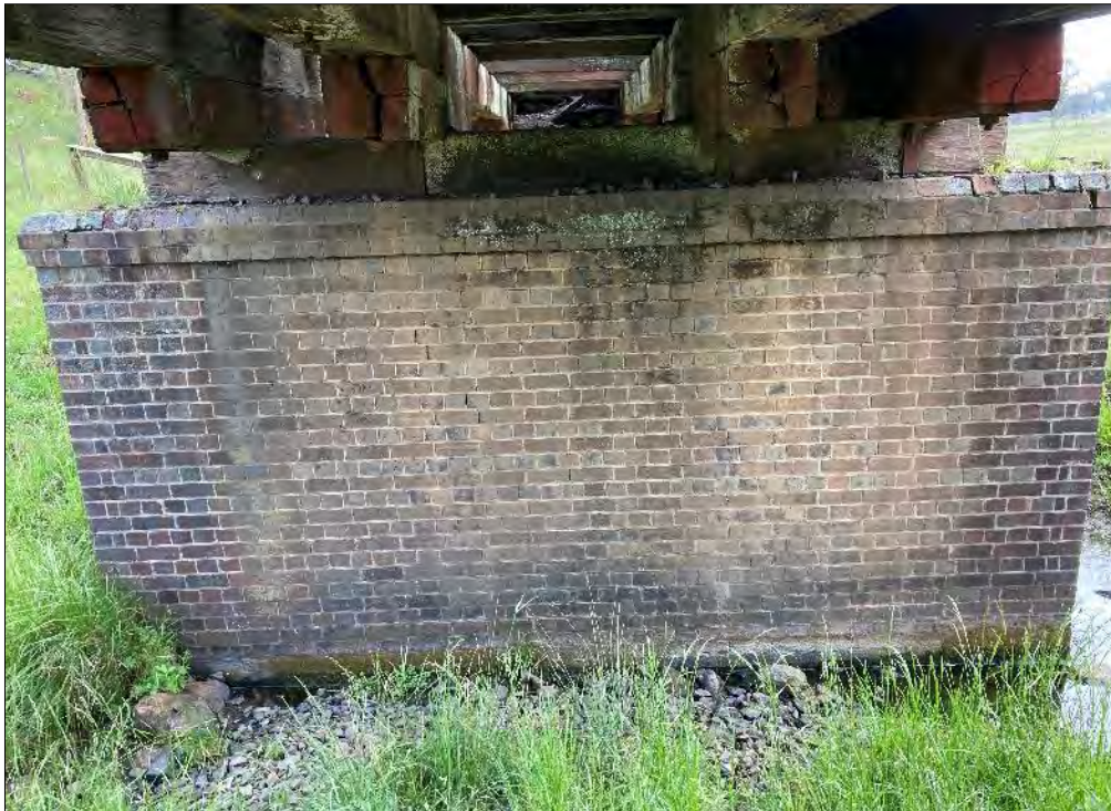
Figure 6-3: View of the brick pier that is approximately 3 metres in height. The timber girders are supported by corbels that rest on a timber cap that bears directly on the brick pier. On either side of the pier there are signs of deterioration and scour. Scour protection (rip rap) is recommended to be installed.
