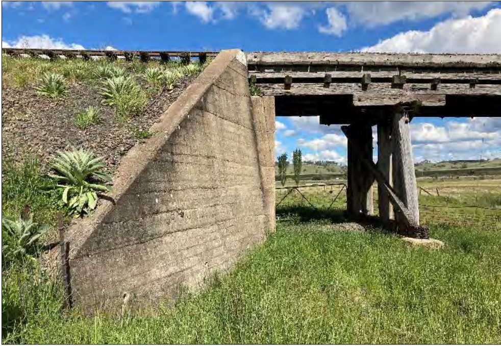
Figure 5-8: View of Abutment 1 which is the typical board-formed, poured place, concrete wing and breast wall configuration. The concrete mass block/seat is in fair condition with the wingwalls intentionally angled back towards the approaches to help overcome the large forces from the approach fill.
