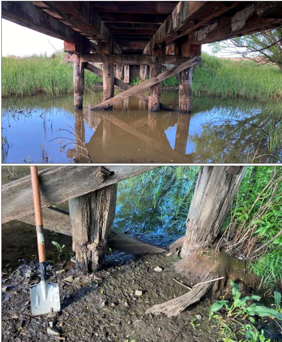
Figure 7-3: View of Pile Bent 2 (top) and Piles 3 & 4 of Pile Bent 1. The bottom of the piles in the ‘splash’ zone are significantly deteriorated with major repairs required. These piles will also require restoration for lateral stability of the bridge. When more than 50% of the piles in the bent require replacing then it is cost effective and beneficial for longevity that the pile bent is replaced with a new frame bent. That is, all piles are trimmed down to bright (solid) wood and a new bottom cap (sill) is placed on top of the pile stubs with the new posts connected to the sill to support the new cap and corbels/girders.
