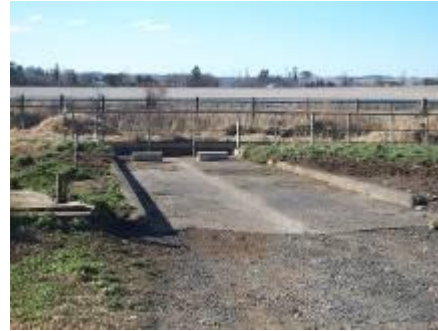
Photos 5 and 6: Truck wash and sediment trap for sales yard
