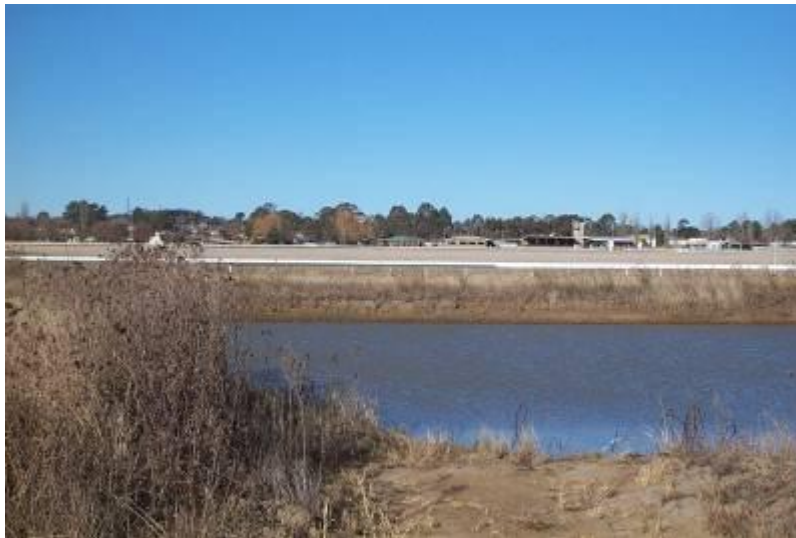
Photo 7: Retention Pond for sale yards high nutrient water to be sprayed on racecourse
