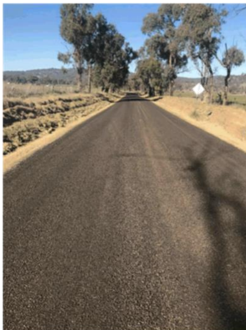
Image 2: Graded Aggregate Seal on Yarraford Road
