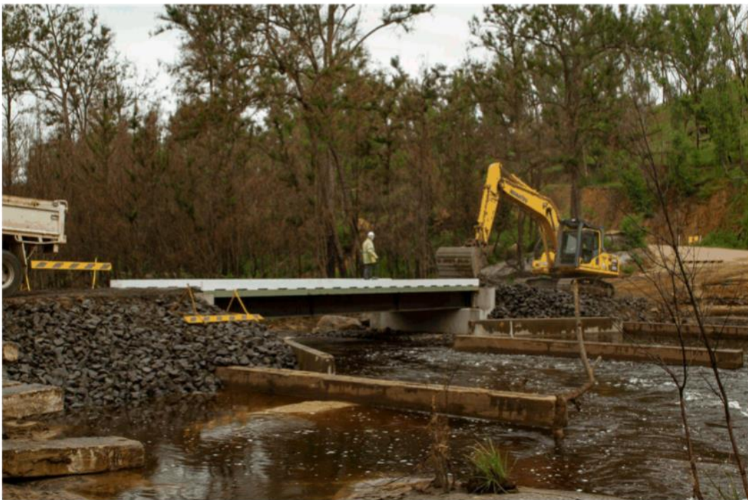
Image 1: Emergency side track installation after Wytaliba bridge was lost through natural disaster (fire)
