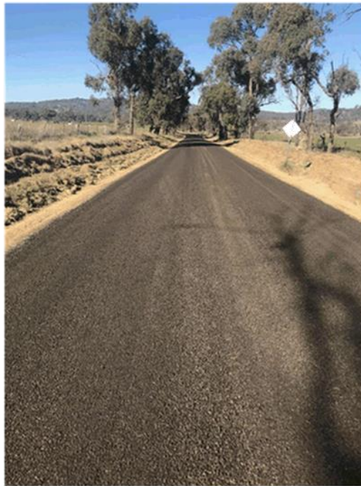
Image 2: Graded Aggregate Seal on Yarraford Road
