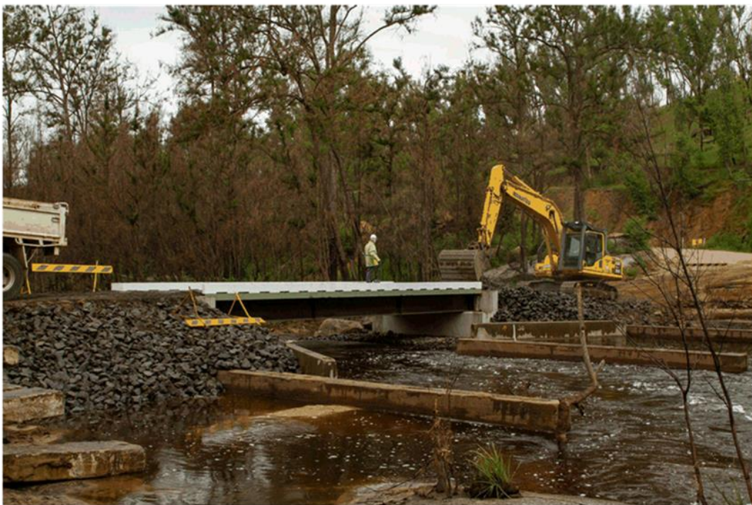
Image 1: Emergency side track installation after Wyaliba bridge was lost through natural disaster (fire)
