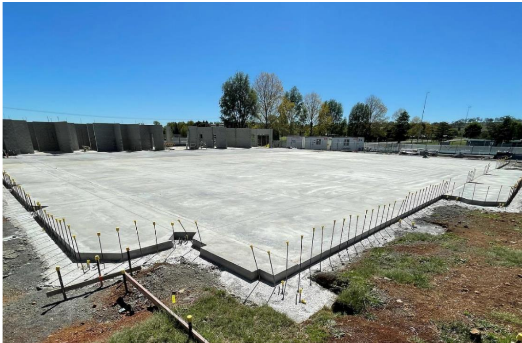
Image 6: Complete Concrete Slab – Warwick Twigg Indoor Sports Complex
