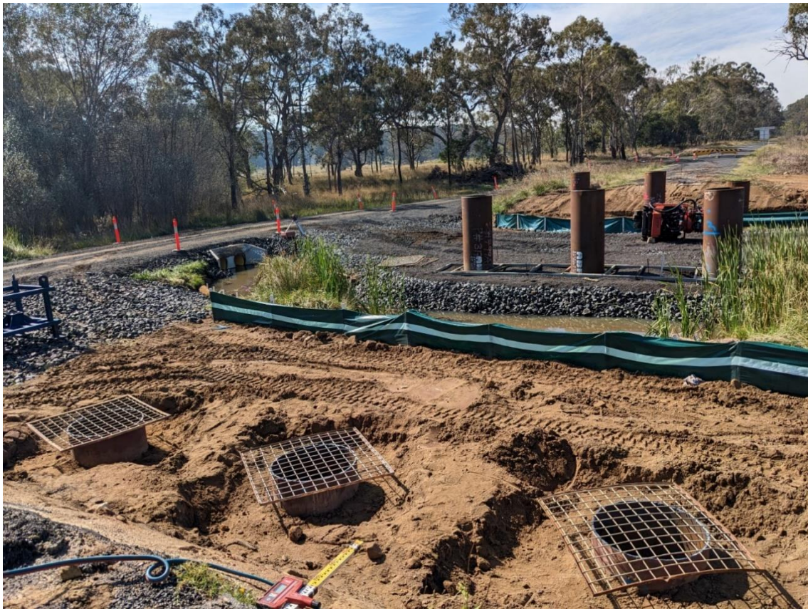
Image 2 – Installing steel casings for new piles
