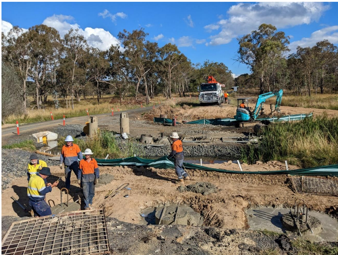
Image 3 – Pouring the concrete piles
