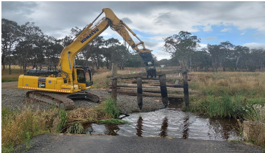
Image 1 - Removal of the old timber piles
