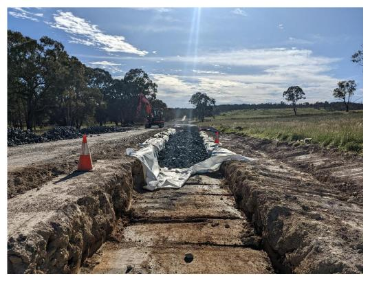
Figure 2: Rock Subgrade Replacement on Bald Nob Road - November 2022
