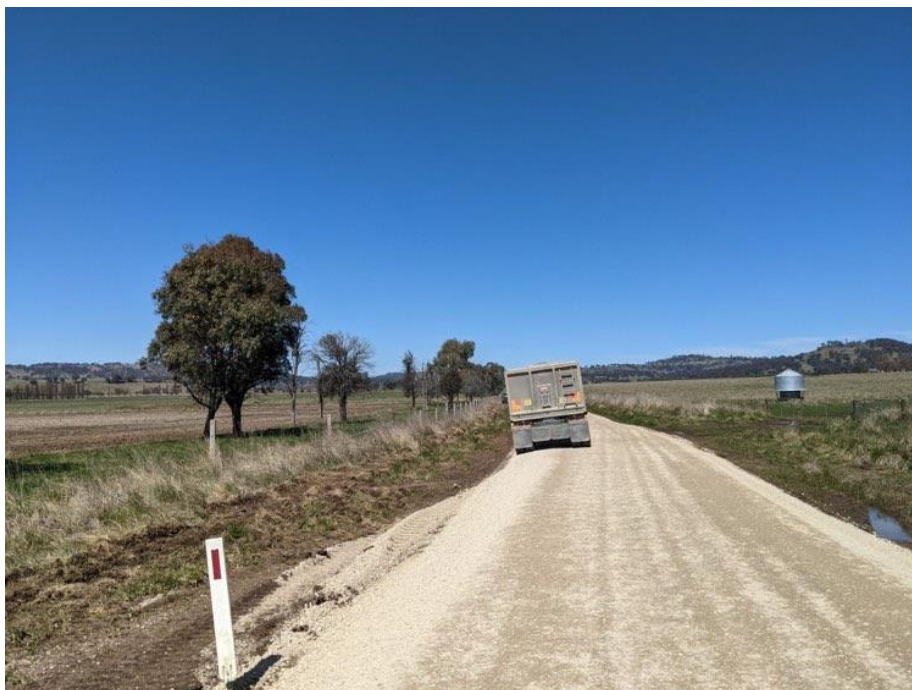
Image 4: Gravel re-sheeting works on West Furracabad Road
