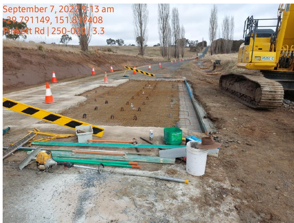
Image 3: Repair of damaged concrete pavement – Pinkett Road – September 2022
