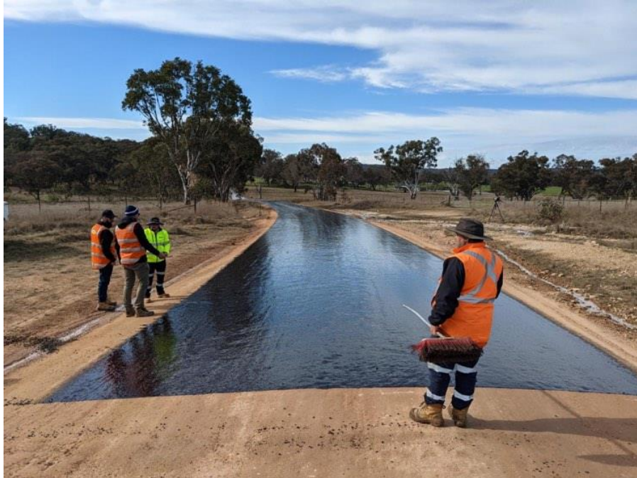
Image 3: Bitumen emulsion sealing trial on Gordons Road
