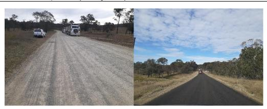
Image 2a and 2b - Completion of the new seal on Pinkett Road
