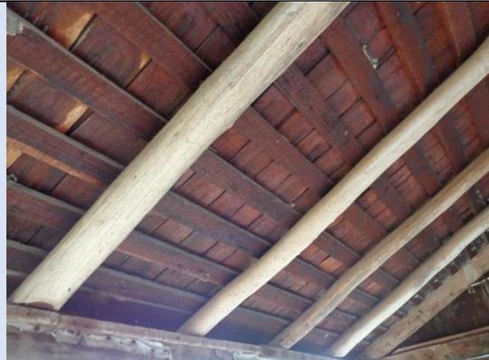
Close batten spacing is also another indicator of a former shingle roof.
